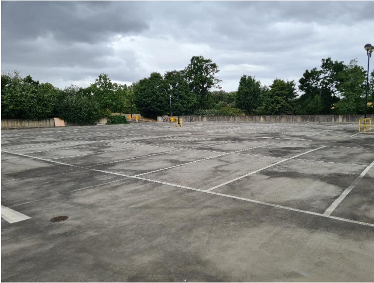
Plate C.1 Upper floor of the on-site car park.
