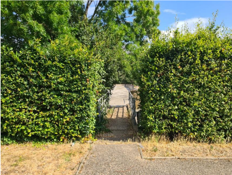
Plate C.2 Pedestrian access bridge connecting the road to the upper level of the car park.
