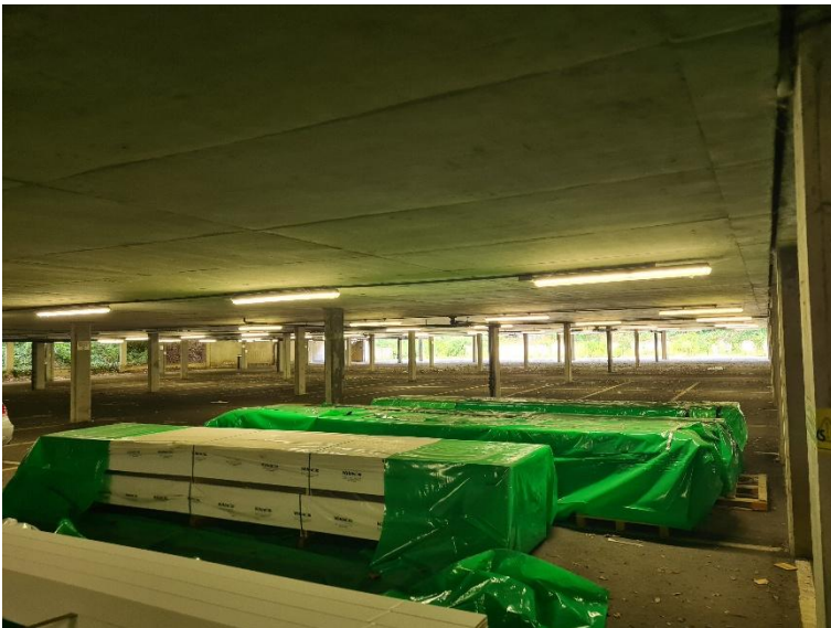
Plate C.3 Material storage and artificial lighting within the lower level of the car park.
