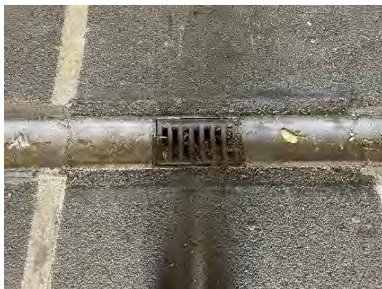
Photo 15: Partially silted up drain located on bottom floor of site
