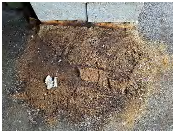
Photo 13: Evidence of historic leaks/spills below fuel storage
