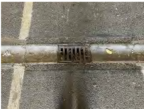
Photo 15: Partially silted up drain located on bottom floor of site
