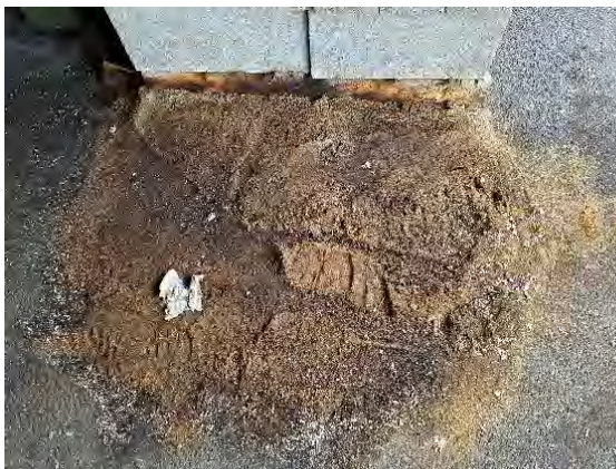
Photo 13: Evidence of historic leaks/spills below fuel storage
