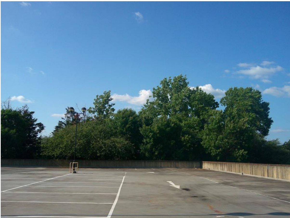
Figure 9: Looking north towards the northern aspect of the car parking structure at the upper level, showing T14 (centre-right) as a point of reference.
