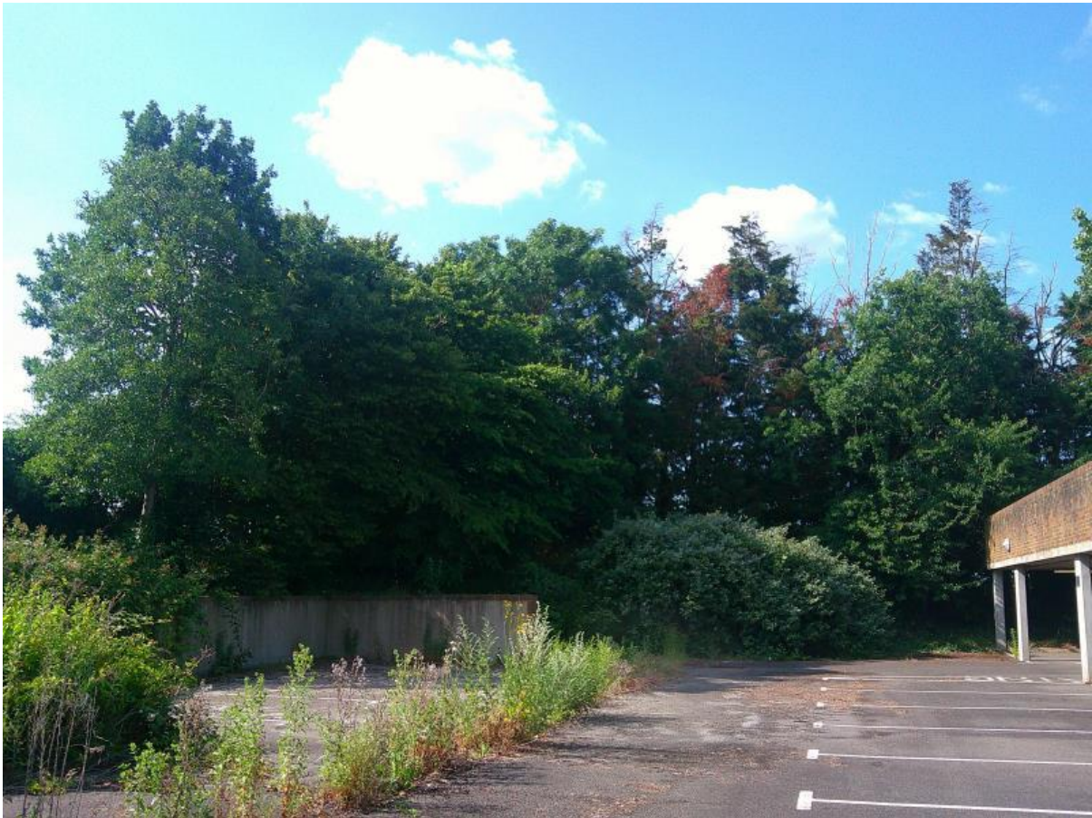
Figure 6: Looking towards the trees to the north-west of the car park structure.
