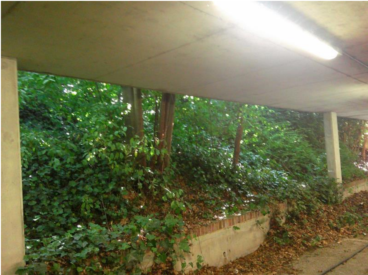
Figure 5: Showing the proximity of surveyed trees to the existing car park structure's southern aspect.
