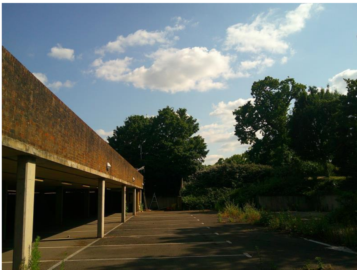
Figure 3: Looking south towards the south-western corner of the Site to the west of the multi-storey car park, showing T114 and T115 (front centre) and T118 (far centre-right) as points of reference.
