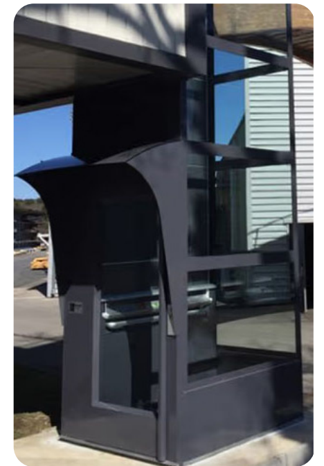
Proposed platform lift, simple discreet design with rain protection to the access level, proposed colour is green
