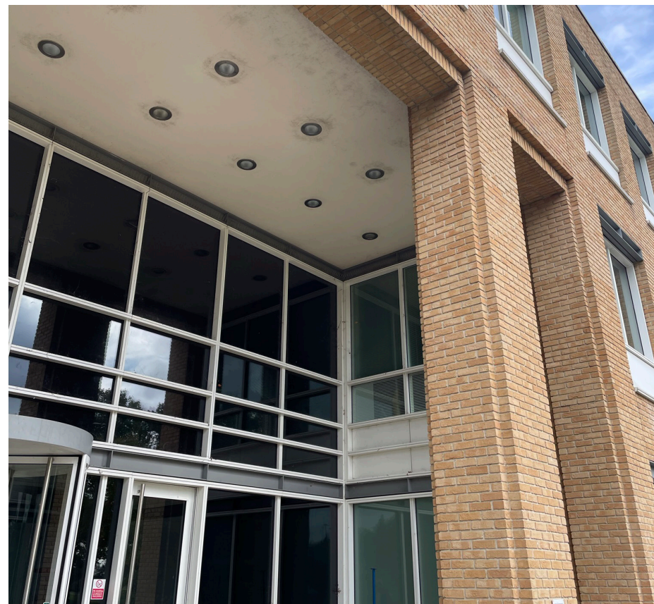
Existing curtain wall to be replaced with solid cladding
