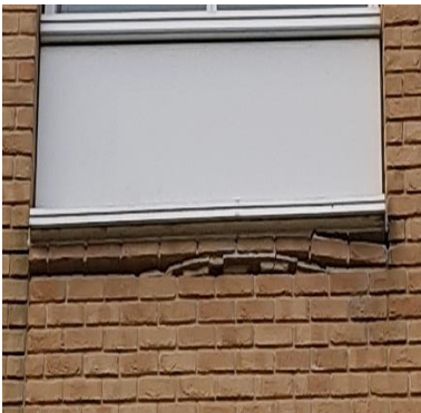
Figure 2.2 Damaged brickwork under a window on the main building.
