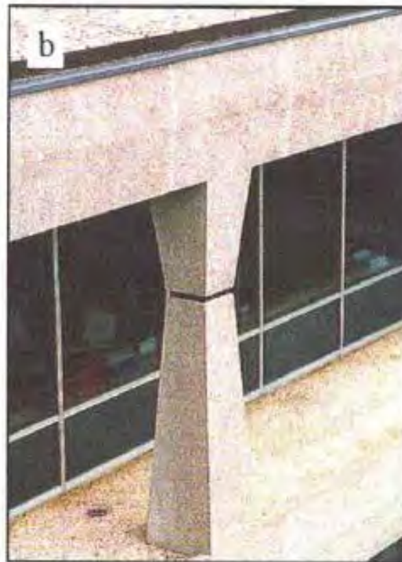
Concrete staining that was noted by Concrete Quarterly in 1988
