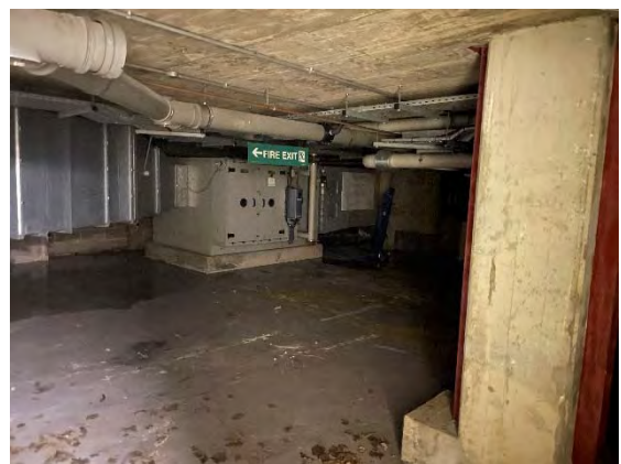
Photo 8: View of basement (plant room) of Hayes Park Central and localised flooding
