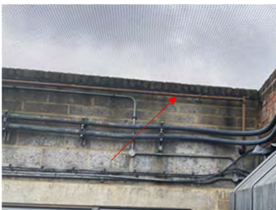
Photo 19: Tank fuel line routed along top of compound
