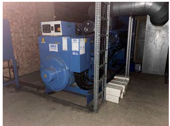
Photo 18: Back up generator with 1,000 litre daily service fuel tank
