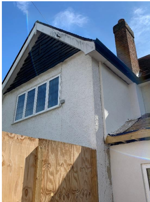
Figure 3 Section of Insulated Render
