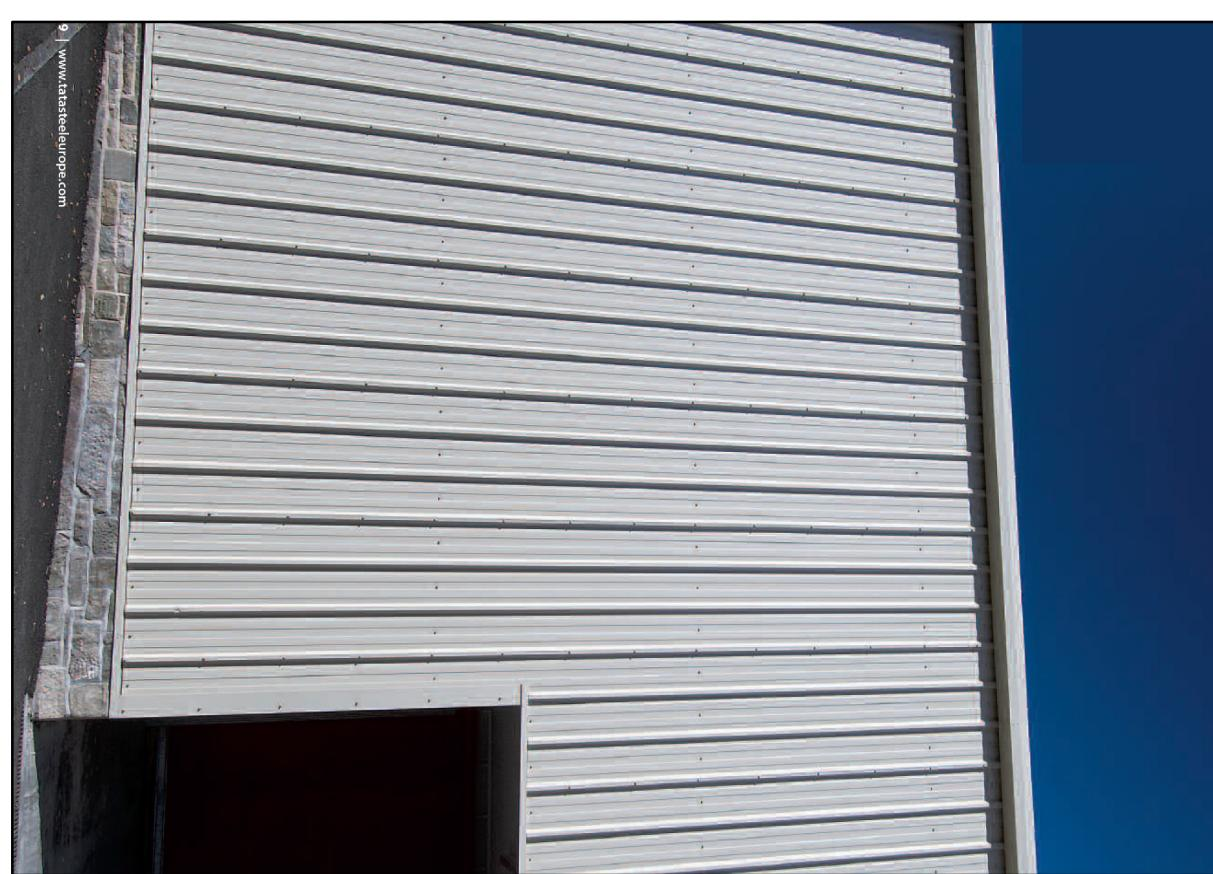
New external walls. Profiled 80mm insulated Tata Steel Trisomet Cladding panels with black metal face.
