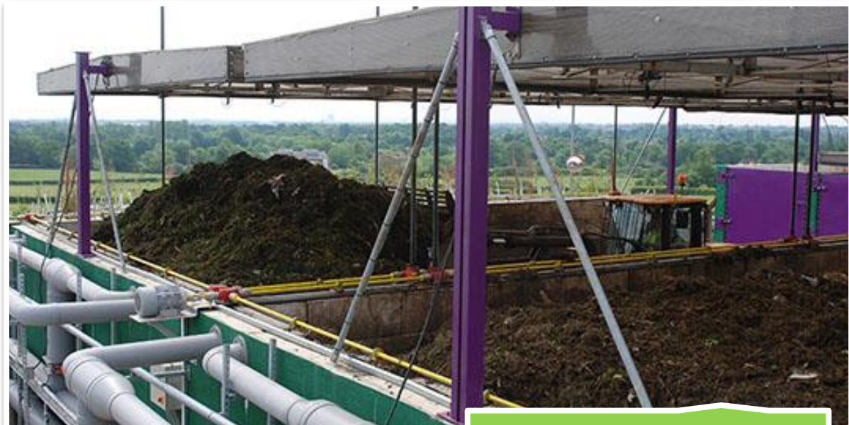
Harefield Composting Facility
