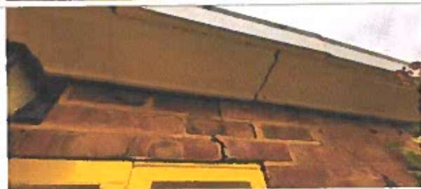
Photograph 12 View of the cracking above the front door.
