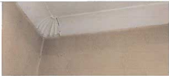
Photograph 30 View of the high-level cracking to the coving in the front bedroom.
