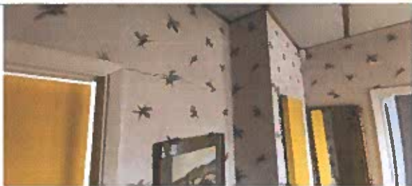
Photograph 19 View of the cracking to the internal walls in the hallway.
