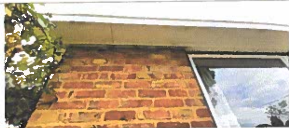
Photograph 9 View of the stepped cracking to the front left corner of the front elevation, at high level.
