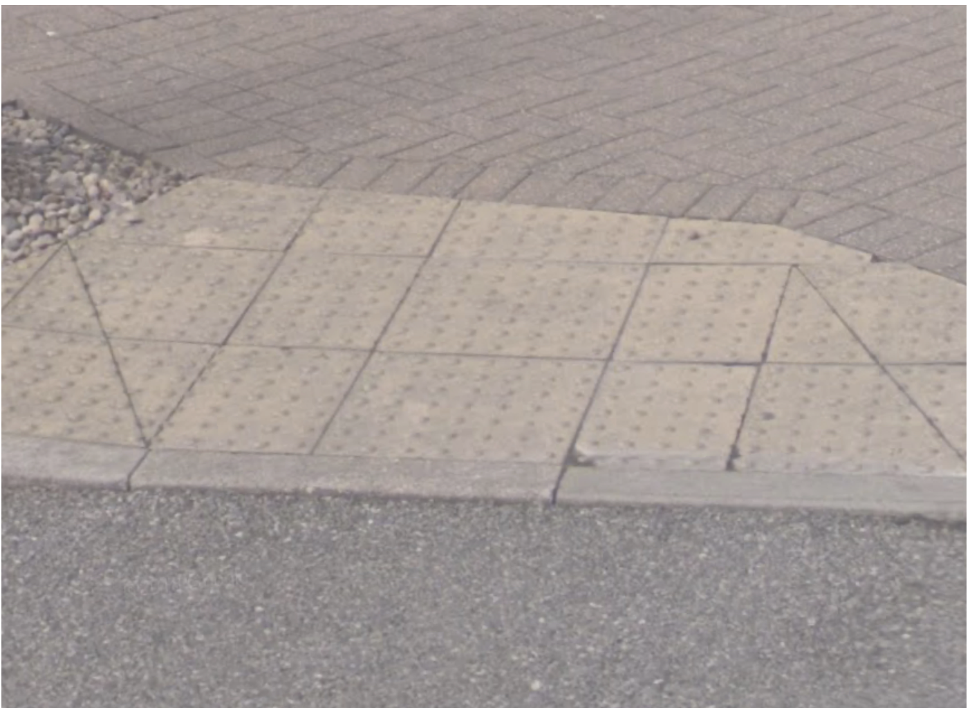
3) Existing Blister Tactile Paving
