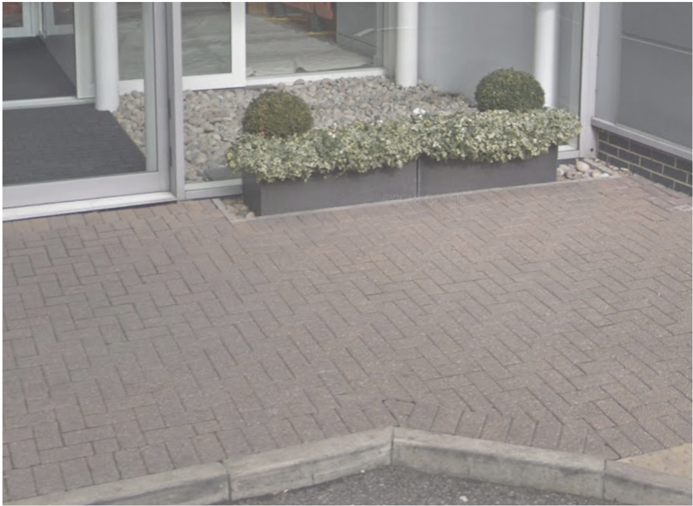
2) Existing Red/Charcoal Block Paving
