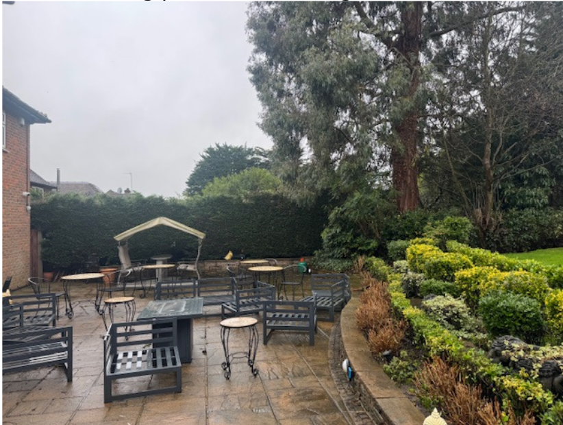
Below: existing patio and retaining wall
