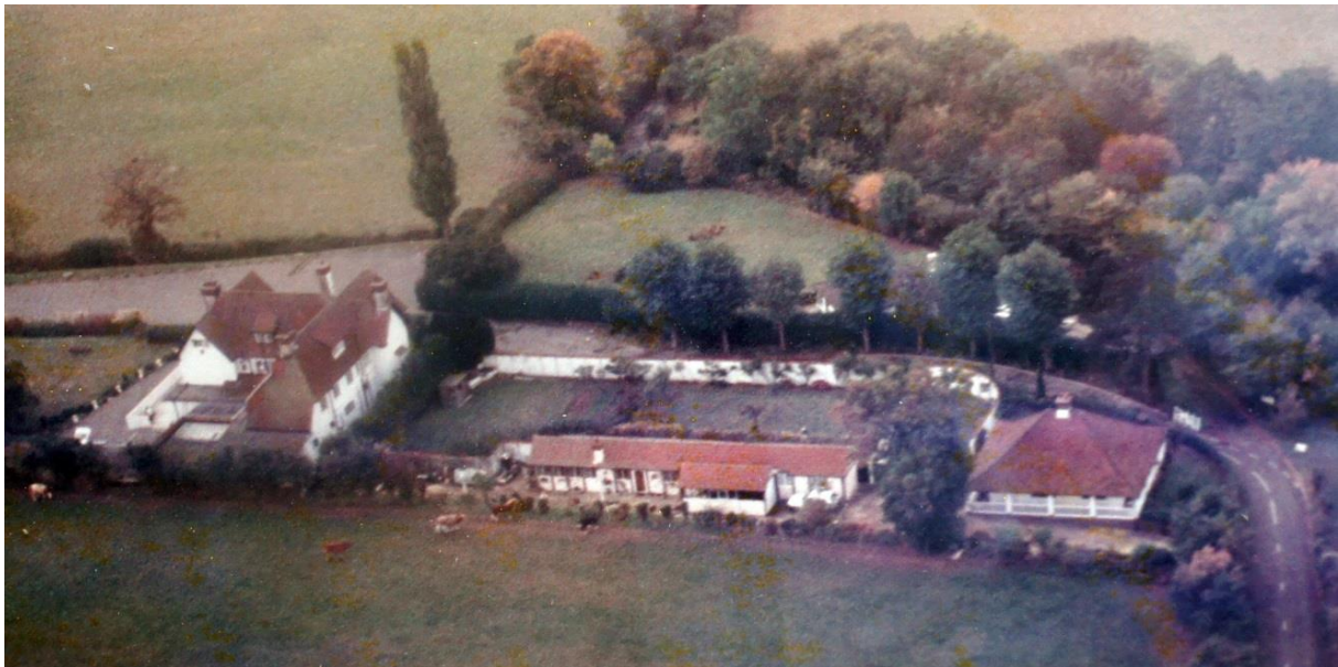
Possibly contemporary photograph of the Group of buildings. Old Orchard Cottage is hidden in the trees.
