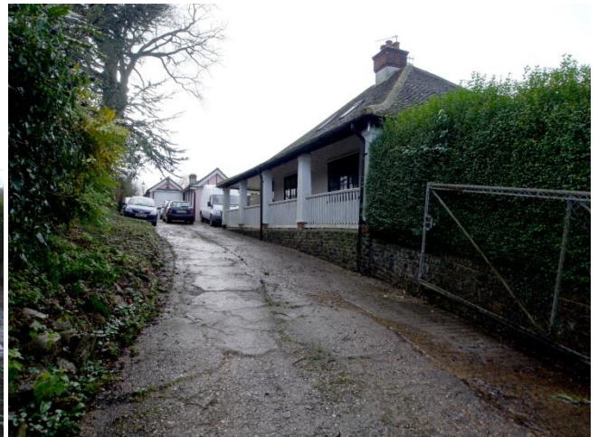
Driveway alongside Old Orchard Lodge Cottage
