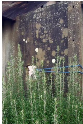
Main cottage construction – rendered no-fines concrete panels within with 'H' section concrete posts. Photo shows the now derelict addition at the south end.
