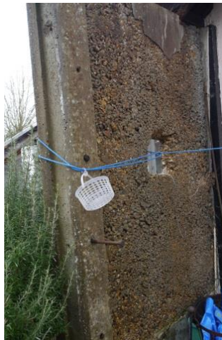
Main cottage construction – rendered no-fines concrete panels within with 'H' section concrete posts. Photo shows the now derelict addition at the south end.
