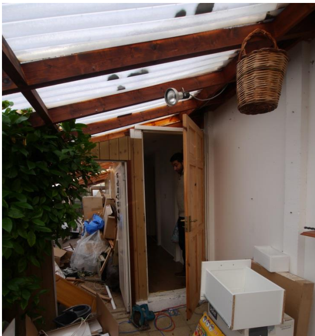
Doorway from crudely built corridor to 'conservatory'
