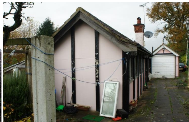
South end and attached garage. Framing of a previous 'extension' is visible in the foreground
