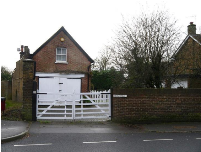
Coach House in Park Lane
