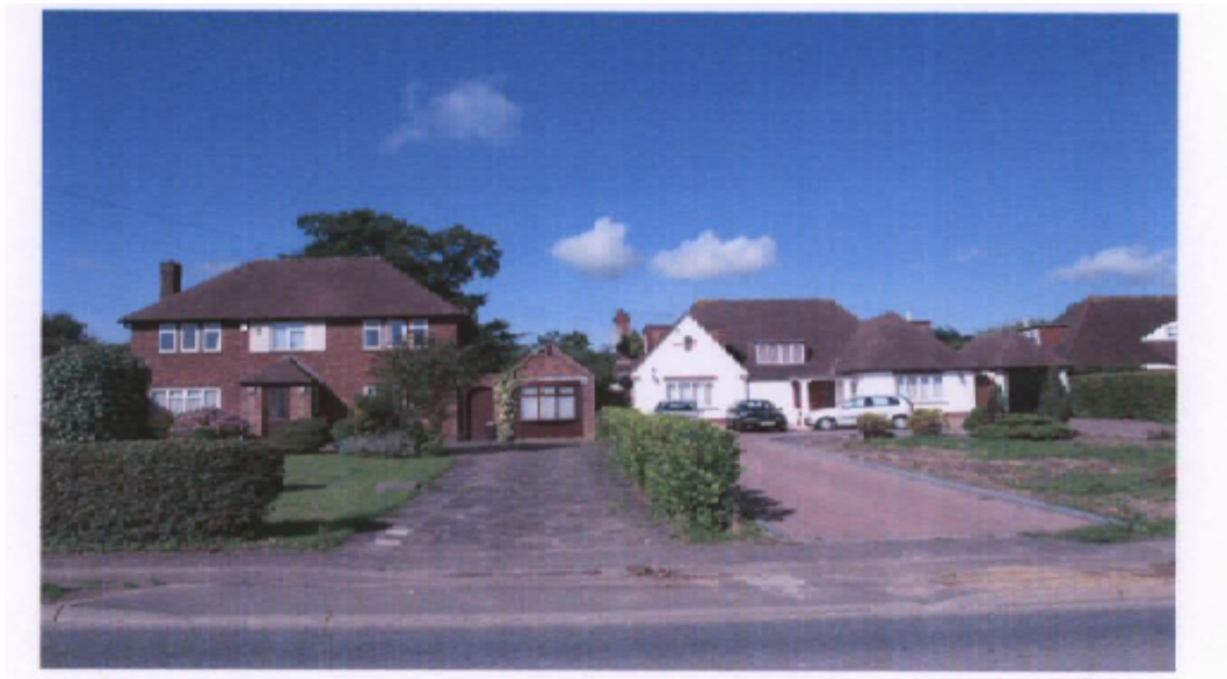
View of the previous house in juxtaposition with its neighbour at No 13. Please note the outbuilding to the right of the premises
