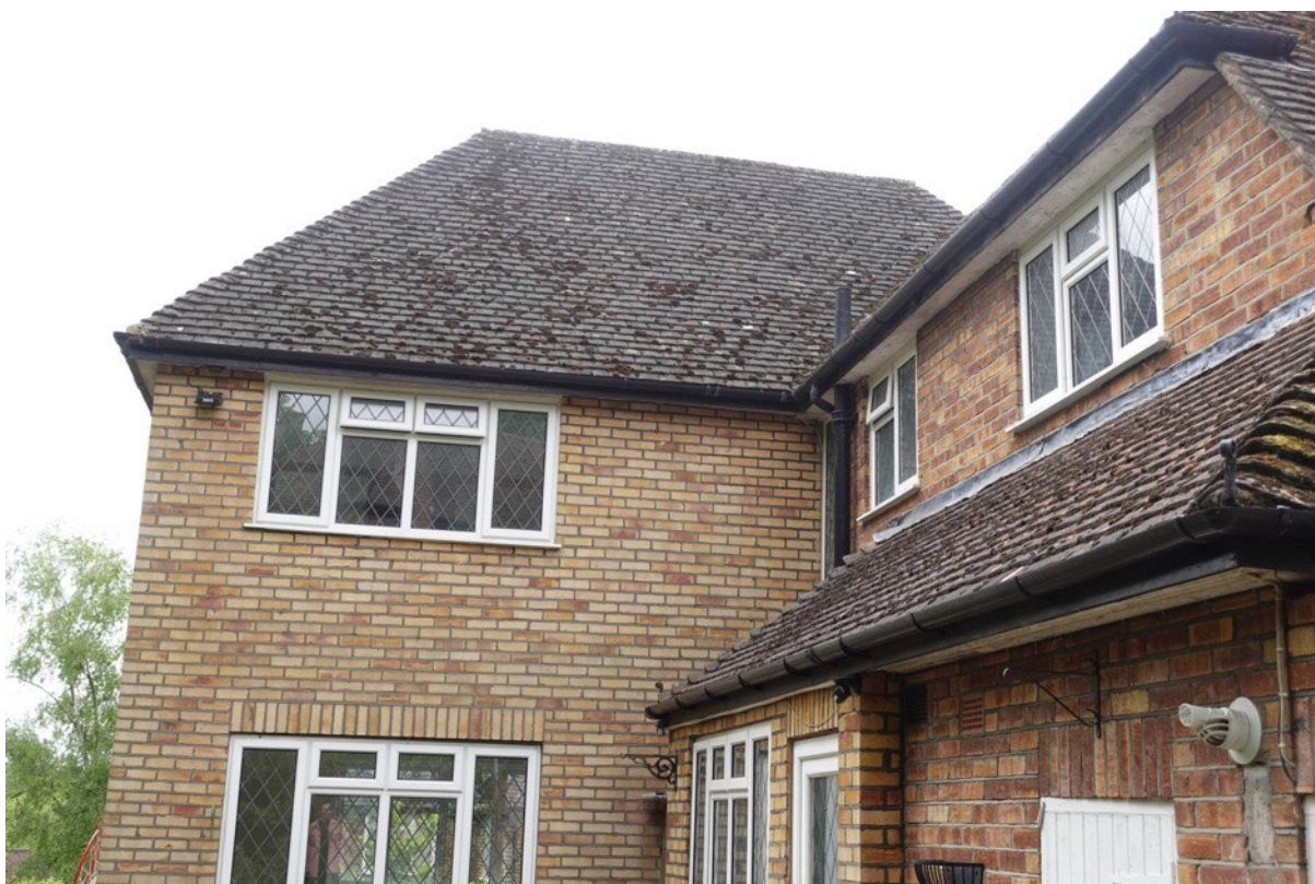
Plate 13: Eastern Elevation – Gaps between roof tiles
