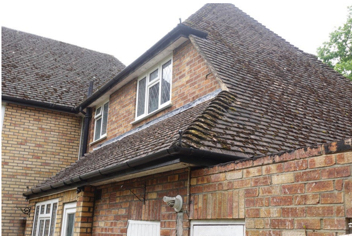
Plate 12: Lifted Roof tiles – Rear (Eastern) elevation
