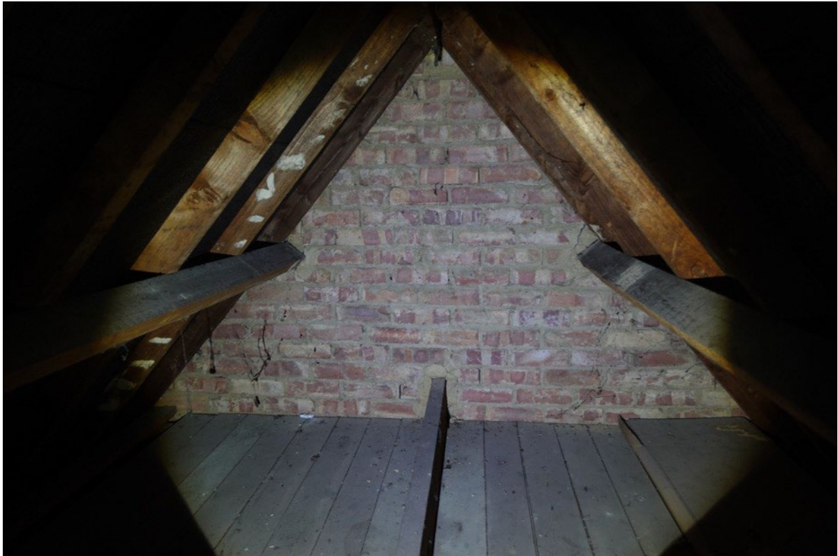
Plate 15: Brick gable end all intact – no entry points noted
