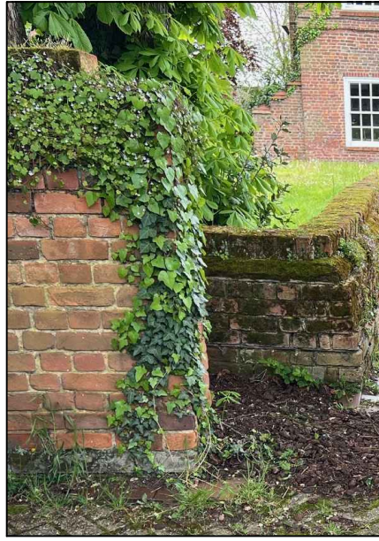
4). Repair required to brick coping with age appropriate bricks and mortar
