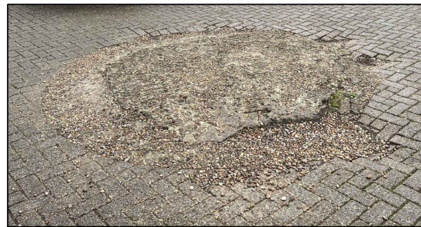
3). Damaged area of block paving to be lifted and relaid. Sub-base and make-up to be same depth as for surrounding block paving
