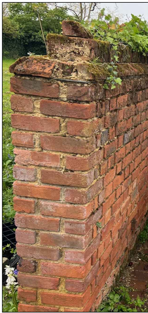
2). Repair required to brick coping with age appropriate bricks and mortar
