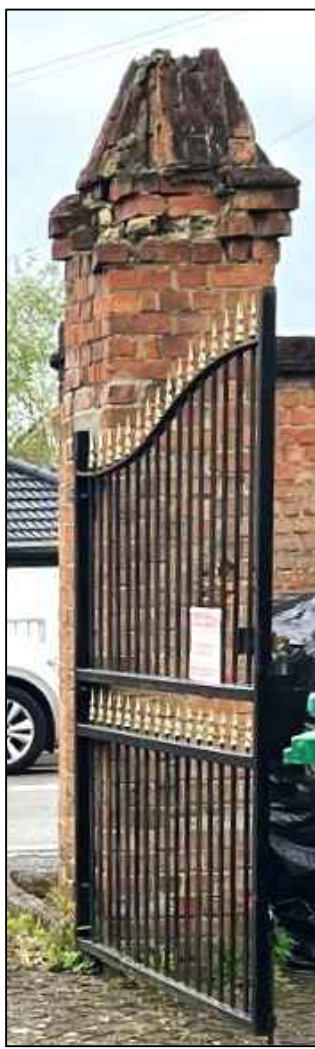
1). Repair required to brick pier with age appropriate bricks and mortar
