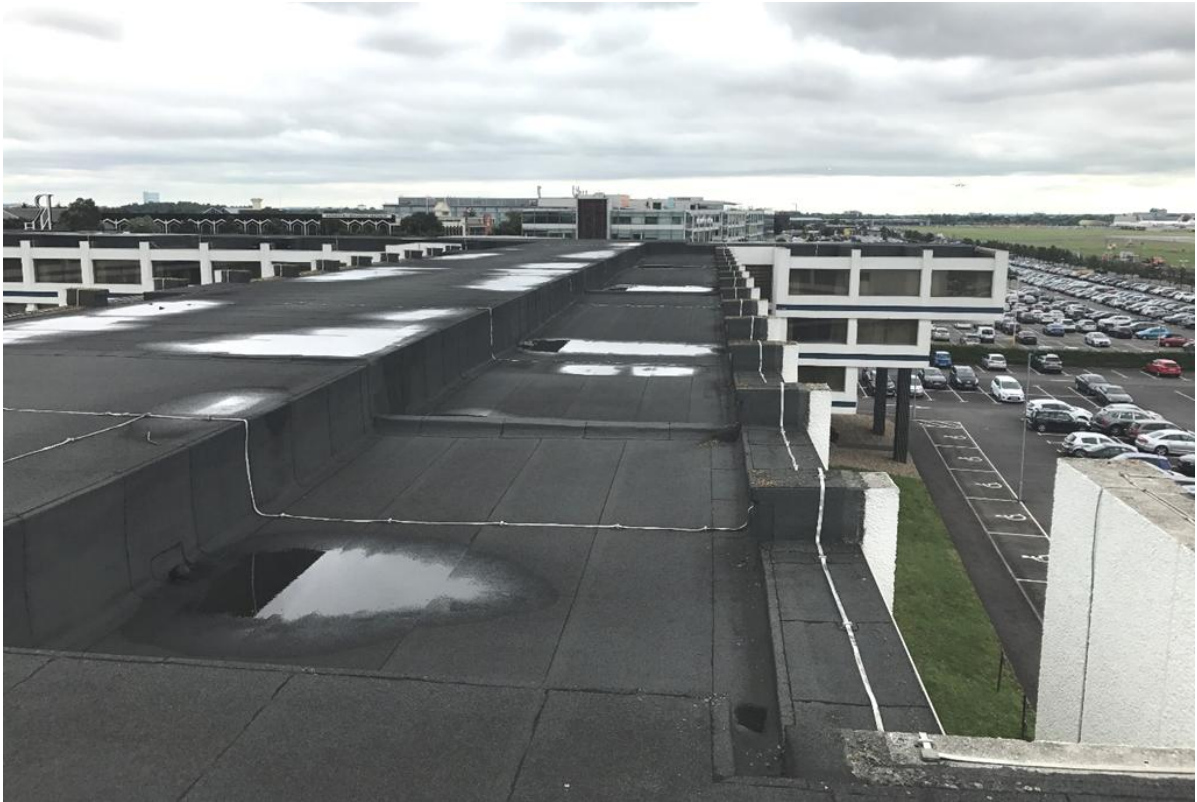
Picture 5 – View of roof facing East. Column lines punctuating the parapet are indicated. Services “top hat” is visible on LHS
