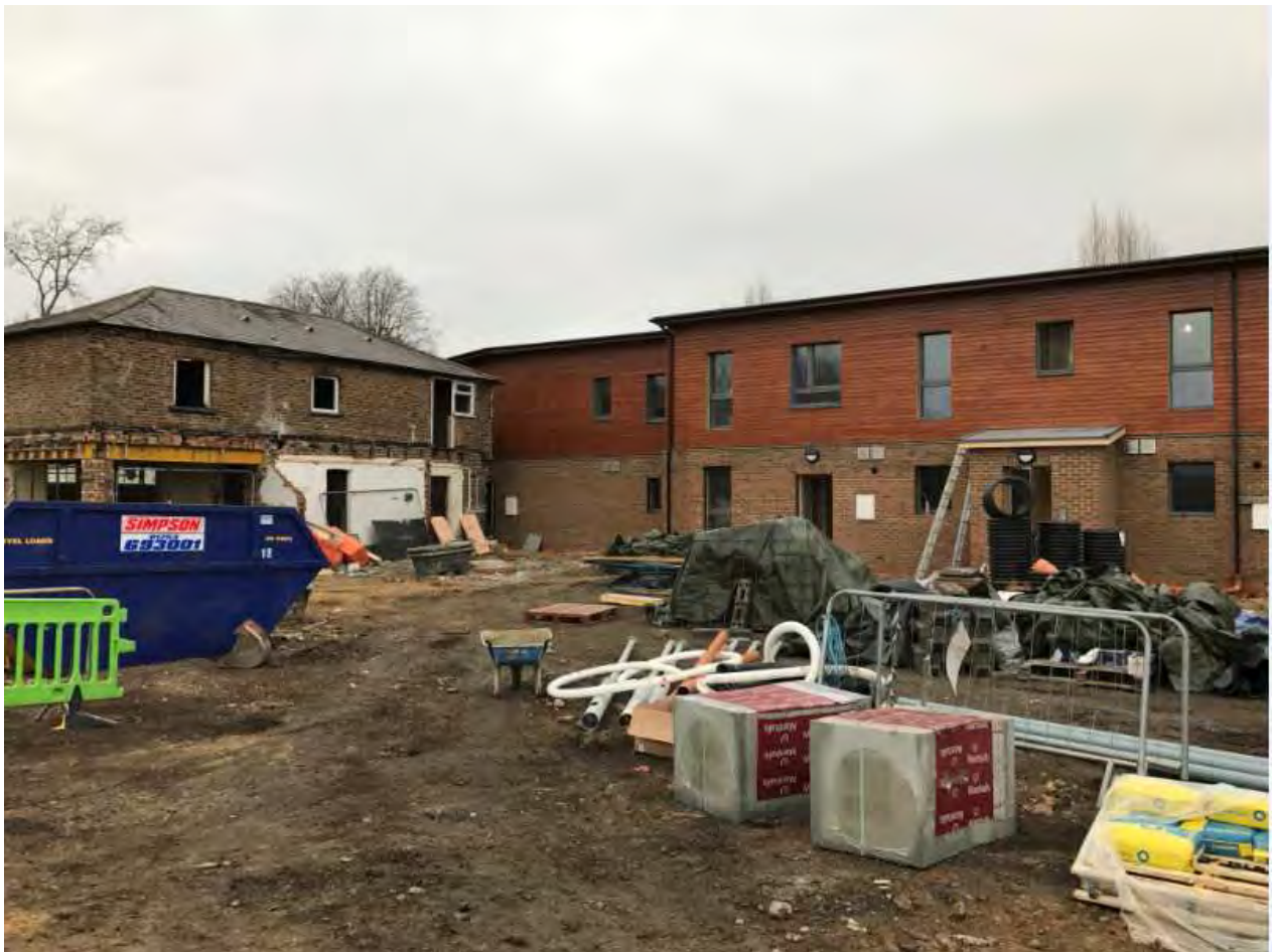
Rear Elevation (December 2016)
