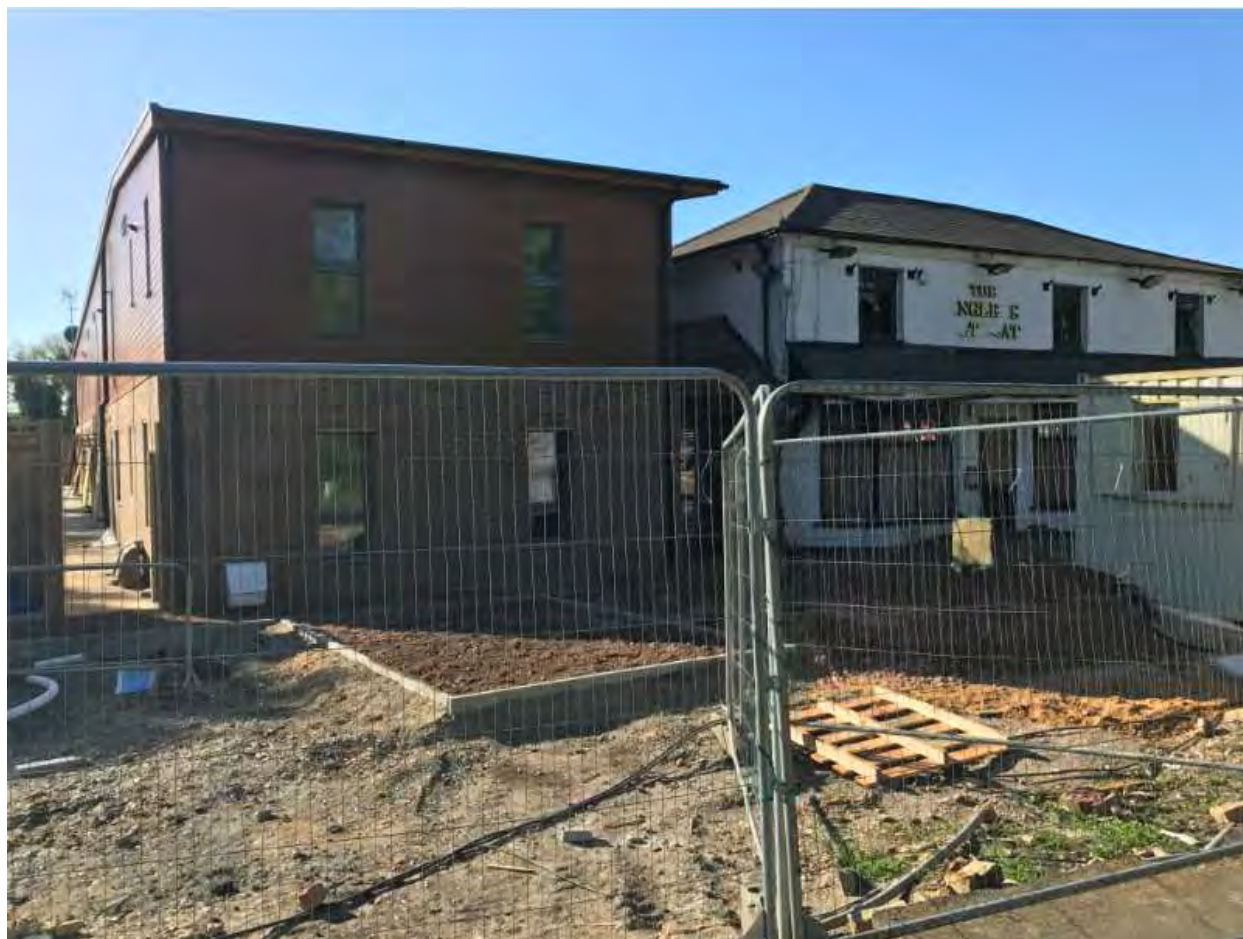
Eastwards view (front elevation) (April 2017)
