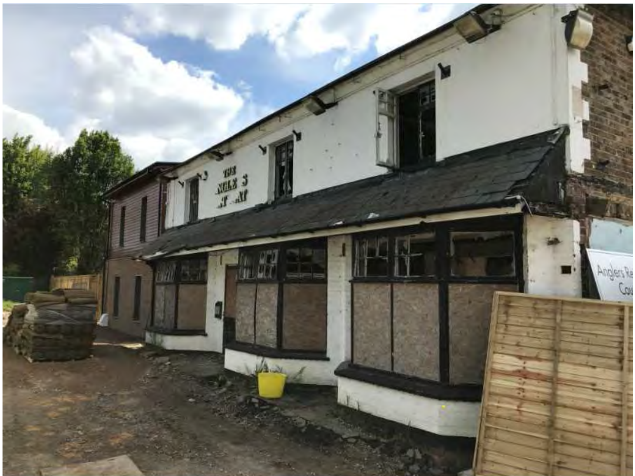
North-east wards view (front) (April 2017)
