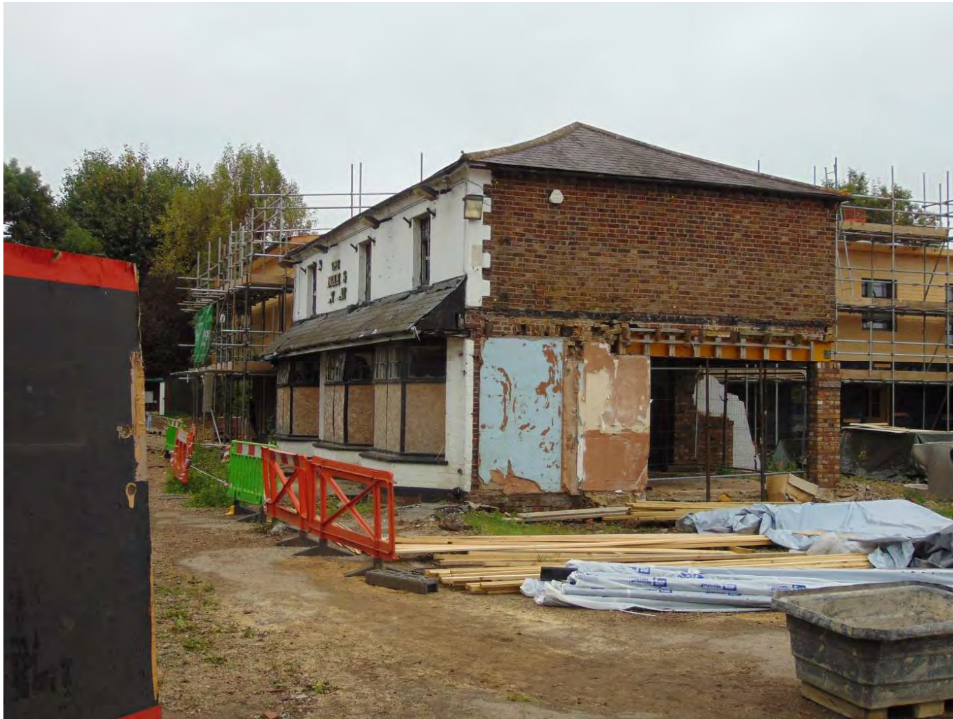
Figure 5 Existing building as it stands in September 2016: extensions demolished and internal space stripped out
