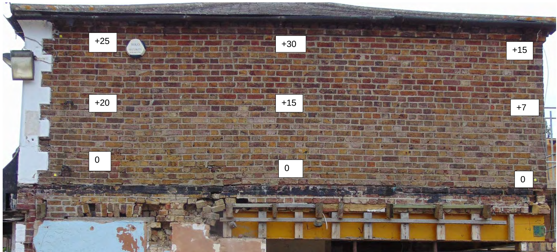
Figure 12 Showing the verticality of the elevation, taken at three set points across the elevation from floor joist up to wall plate
