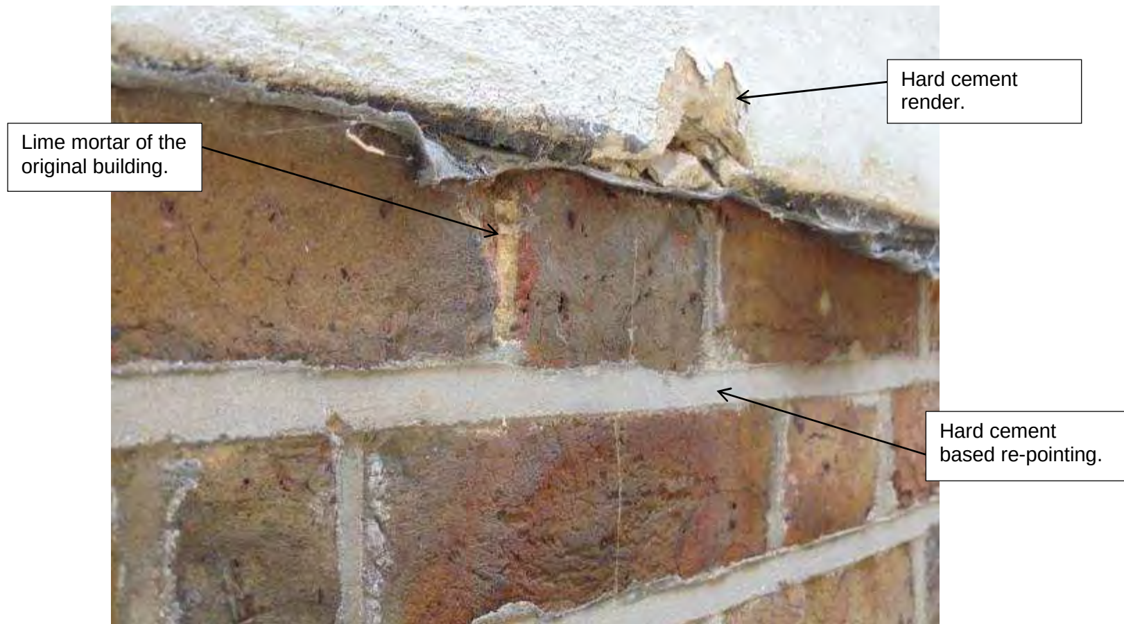
Figure 24 Close up of the original brickwork bedded in lime mortar and re-pointed in a hard cement mortar
