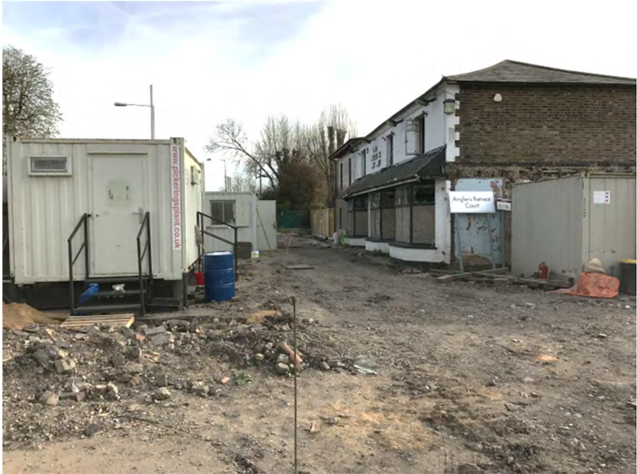
View 8 – North westwards view (Rear east elevation) (December 2016)
