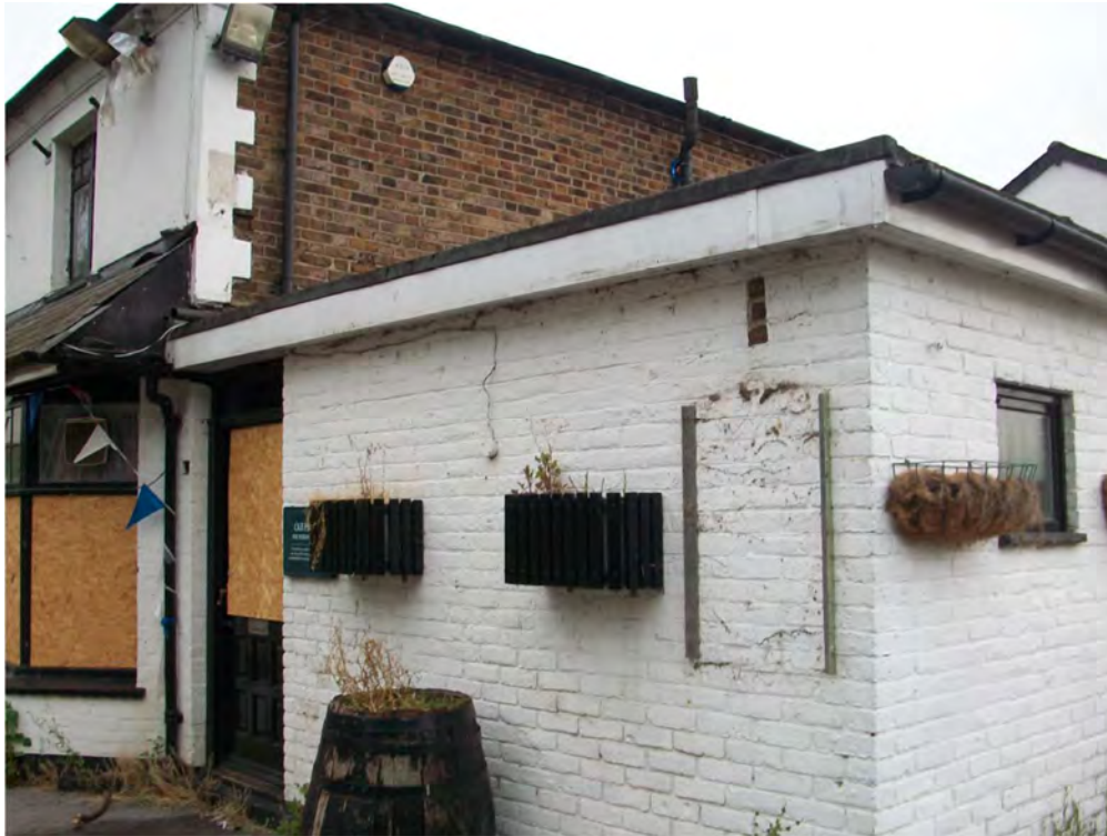
Figure 2-8 Photograph of the modern western extension meeting the original building
