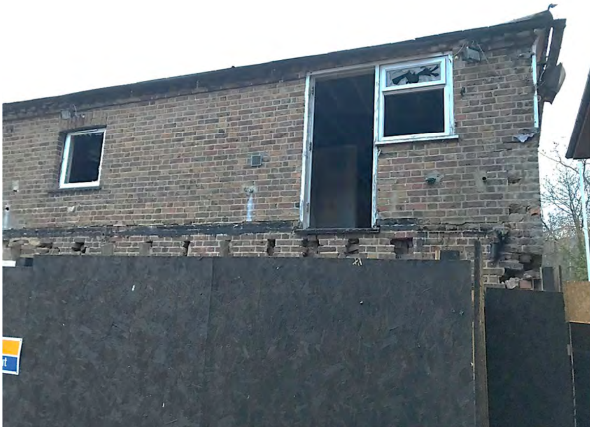
View 11 – Side (south) elevation (December 2017)
