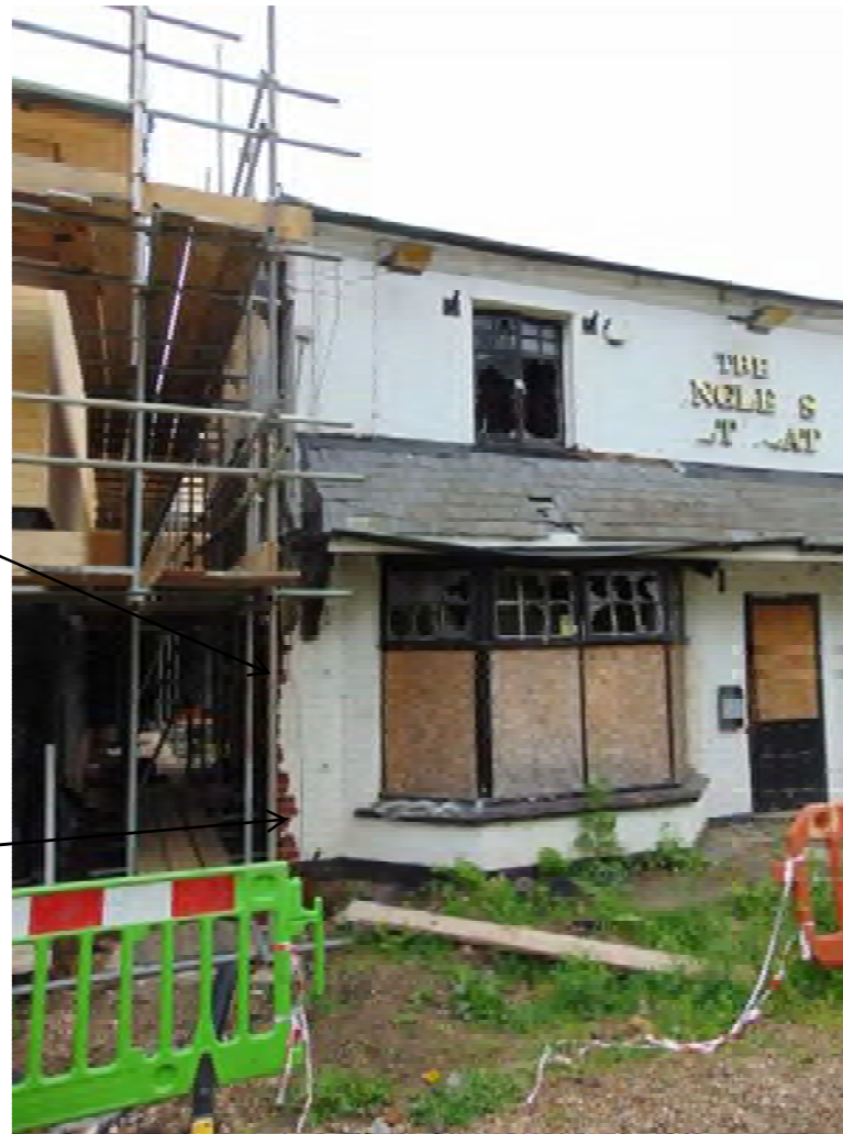
Figure 8 Showing left hand side of front elevation
