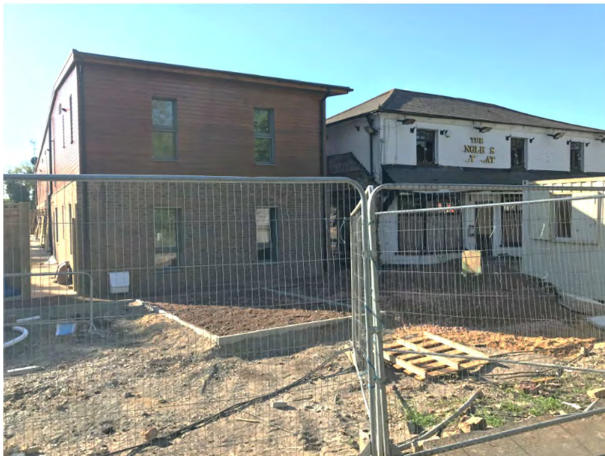
View 3- South eastwards view (front west elevation) (April 2017)
