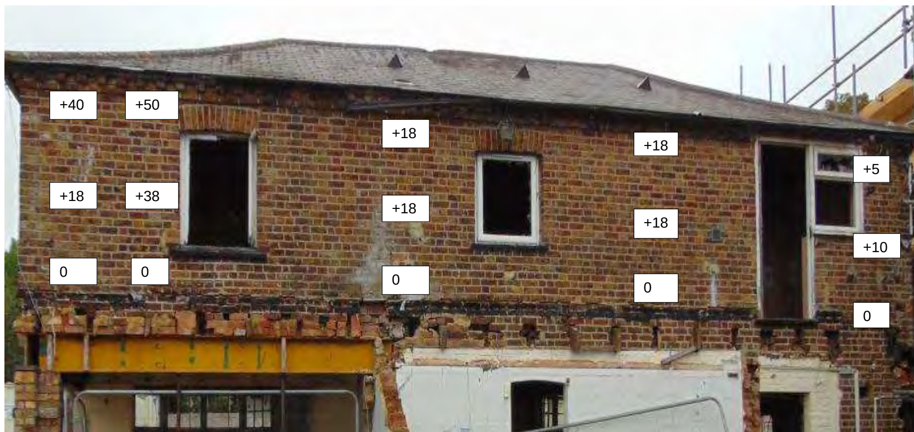
Figure 26 Showing the verticality of the elevation, taken at five set points across the elevation from floor joist up to wall plate
