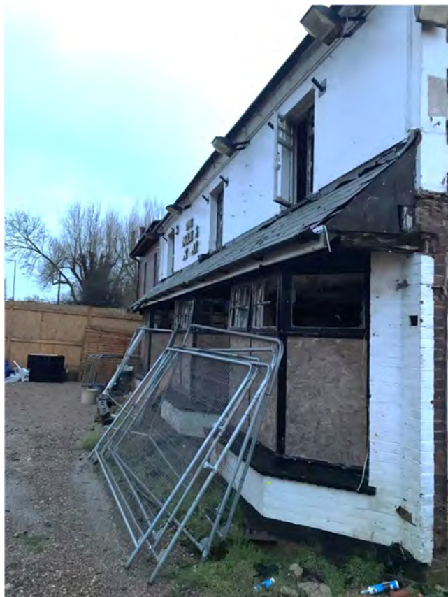
View 9 - Front (west) and side (south) elevation (December 2017)
