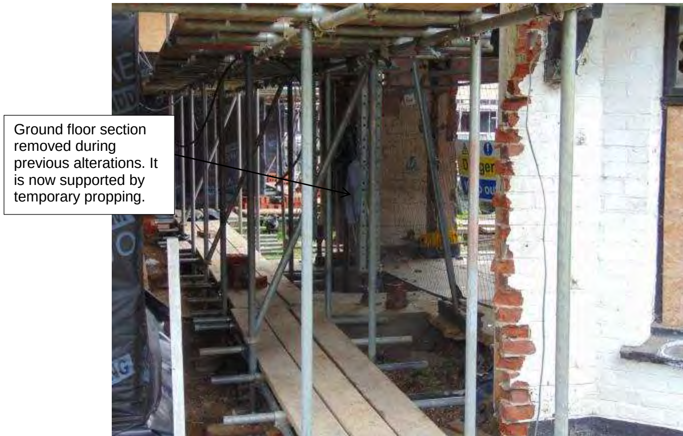
Figure 22 Showing how the first floor of East elevation is supported by temporary propping
