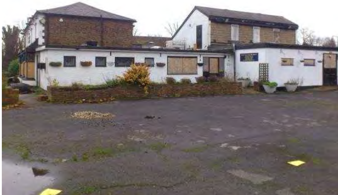
Figure 4 West elevation with extensions (February 2014)
