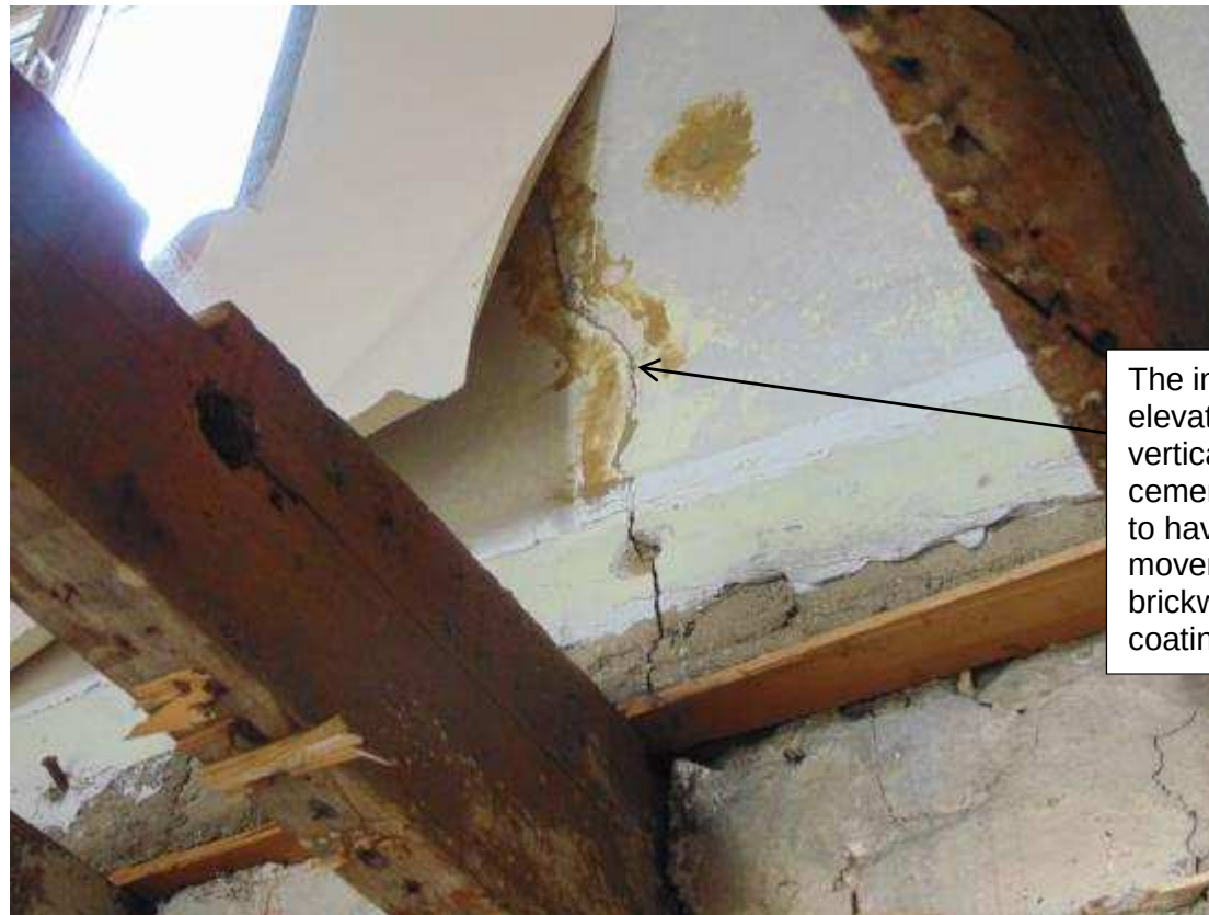
Figure 9 Close up of internal cracking to front elevation
