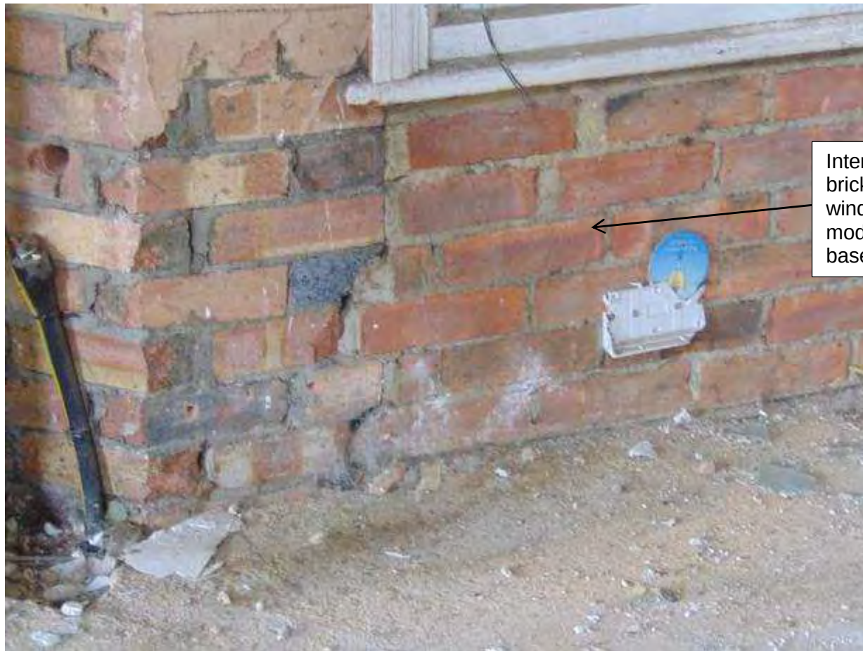
Figure 10 Close up of modern brickwork to bay windows
