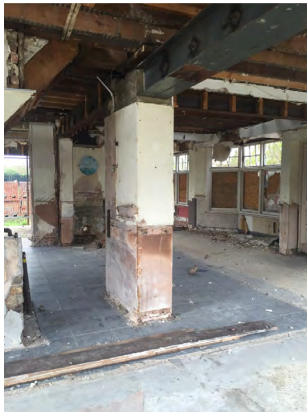
Figure 3: Internal view showing timber floor supported on steel beams and masonry piers
