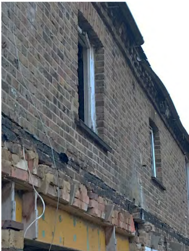
View 11 cont. – Side (south) elevation (December 2017)
