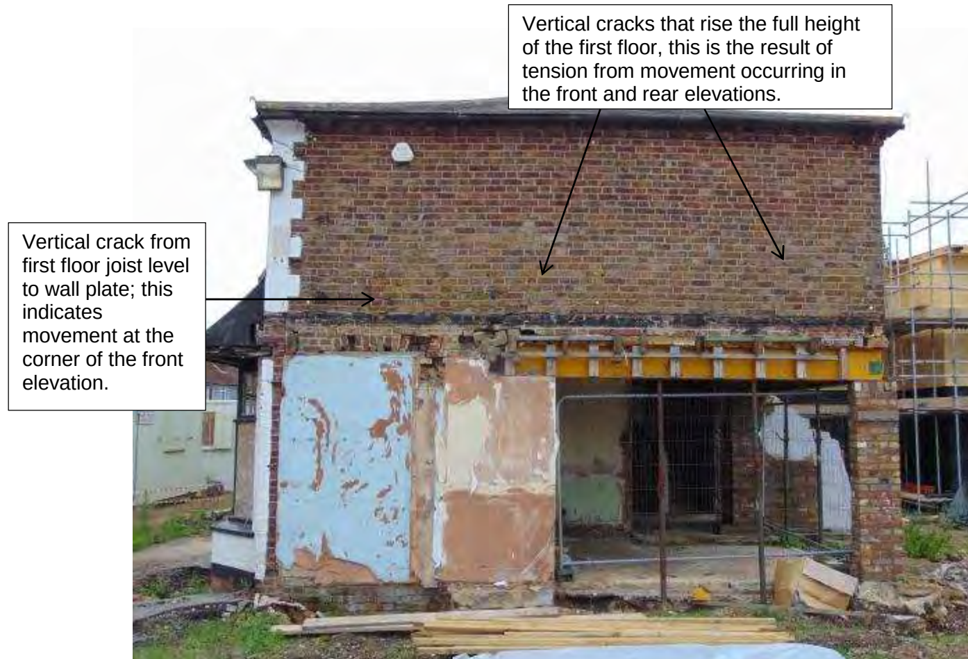
Figure 11 Showing the West elevation
