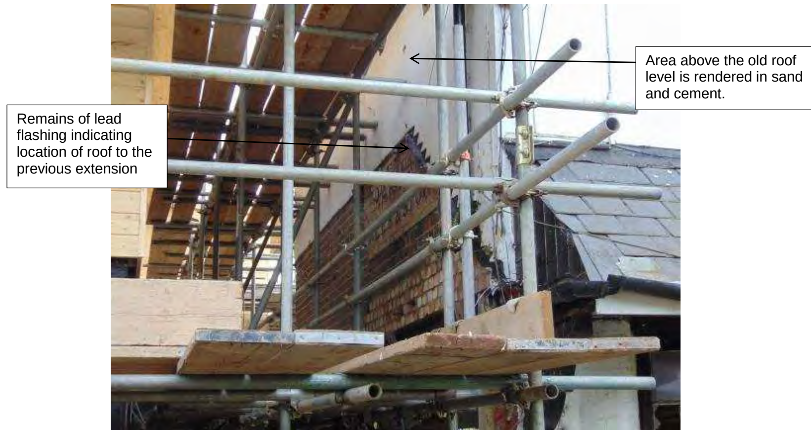
Figure 21 Showing the East elevation and its proximity to the new development
