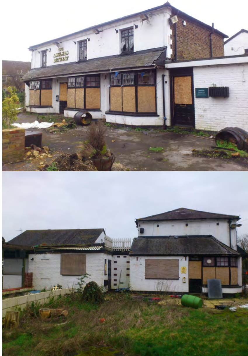
Figure 1: Building with extensions (February 2014)
