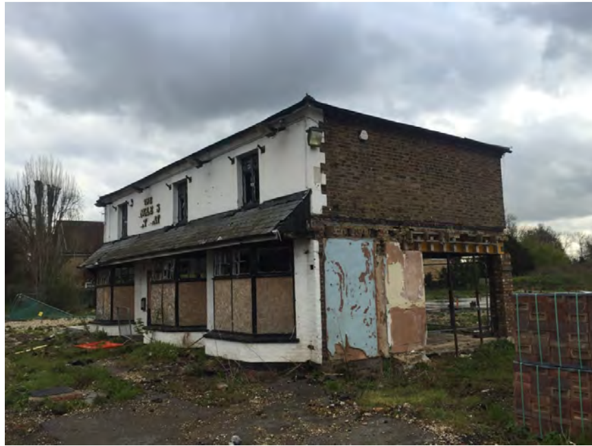
Figure 2: Existing Building following strip out and demolition of extensions
