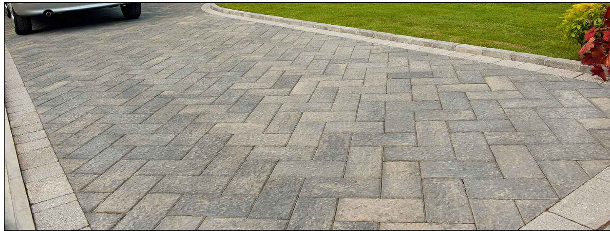
BLOCK PAVING TO PARKING BAYS
