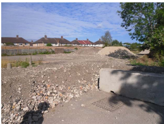
Photo 1. Hardstanding and rubble piles in west of Site
