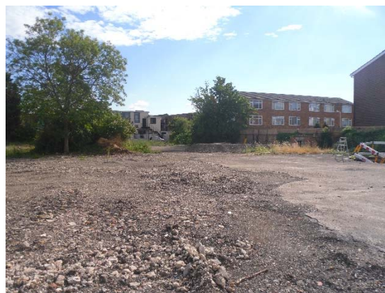
Photo 2. Hardstanding, recolonising ground and trees in east of Site
