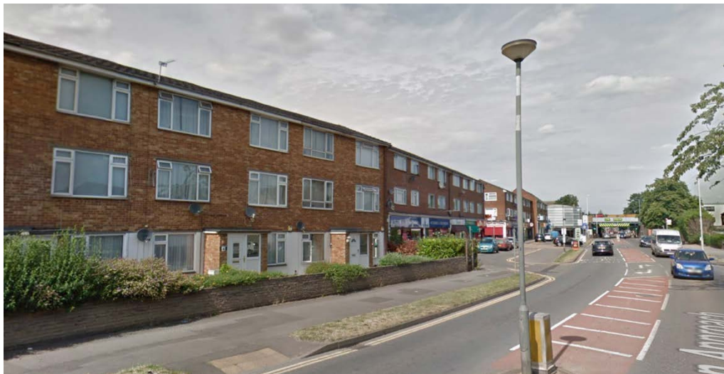
Figure 6: View east along Station Approach towards South Ruislip Station showing the denser three storey development
