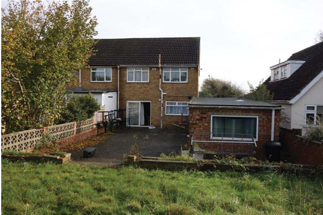
Plate 1: View of site looking east showing house, existing side extension, patio and lawn
