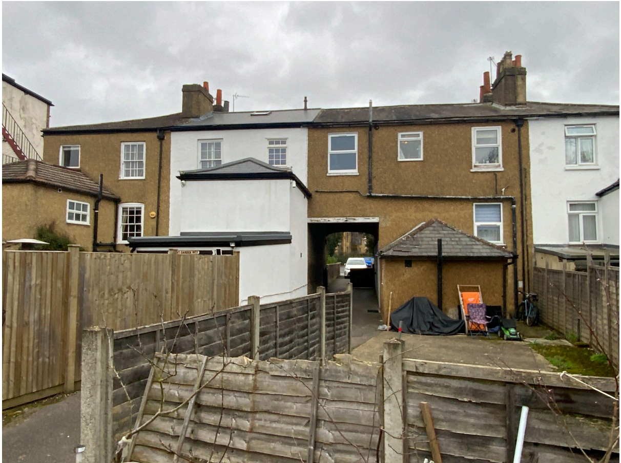
Rear Image of 17A Hillingdon Road, UB10 0AD
