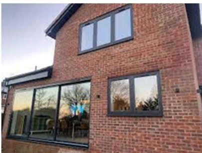
POLYESTER POWDER COATED ALUMINIUM FRAMES DOUBLE GLAZED; COLOUR : BLACK
