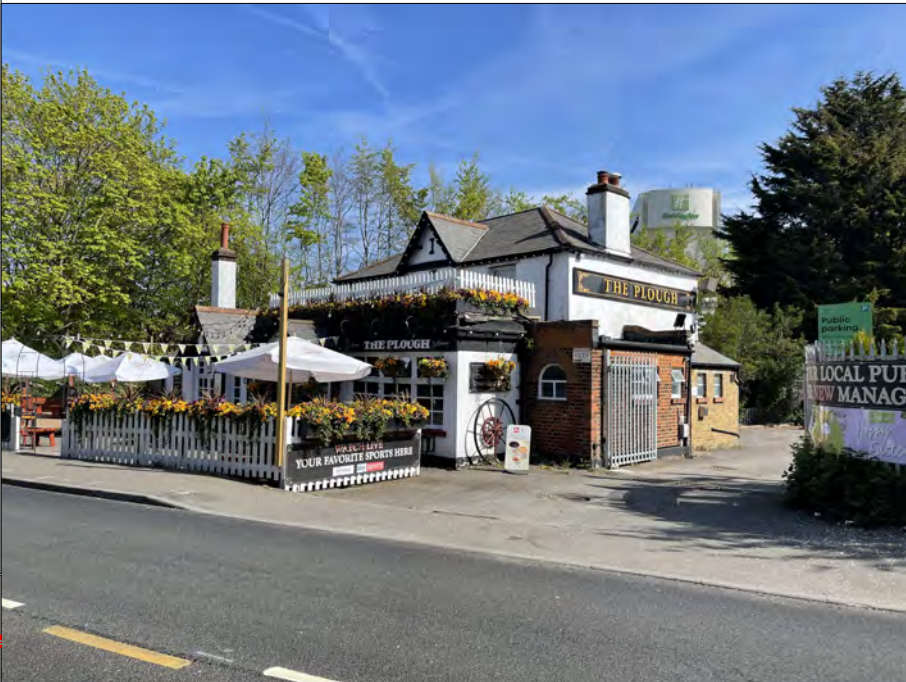
EXISTING SITE PICTURE - SIPSON ROAD
