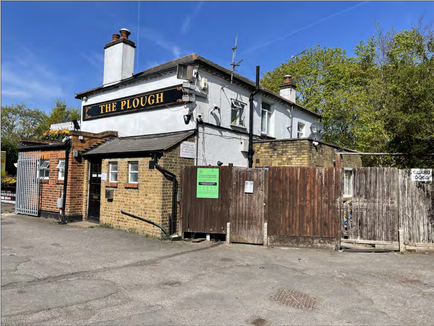
1 1 EXISTING REAR SIDE VIEW 03
