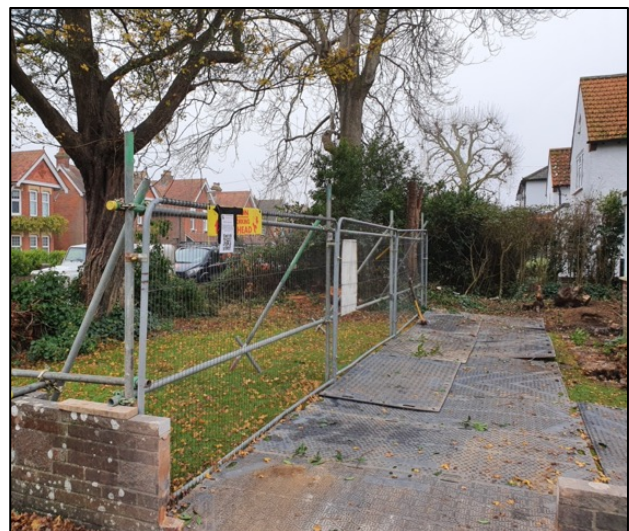
GP2: Tree protection barriers & trackmat ground protection
