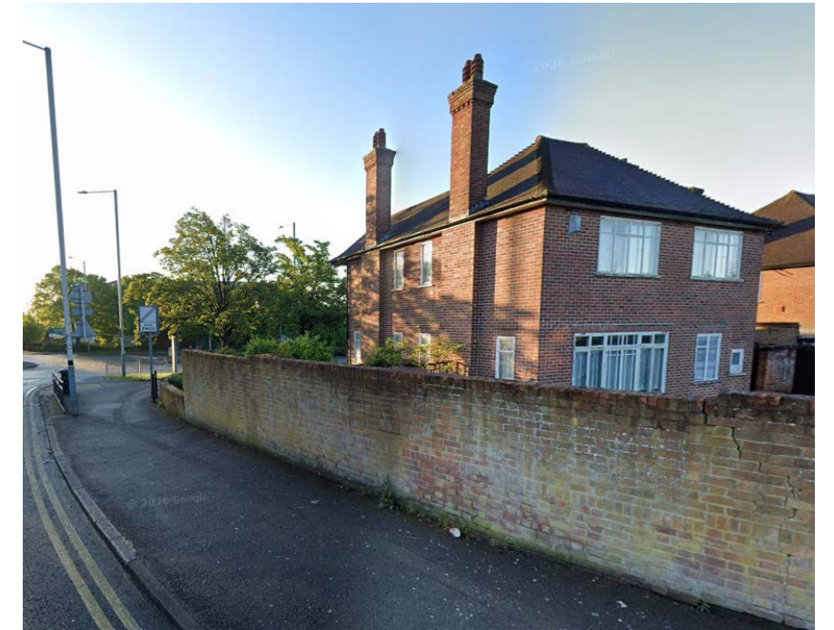
Figure 3.11 Belmont Road Source: Google Streetview May 2021
