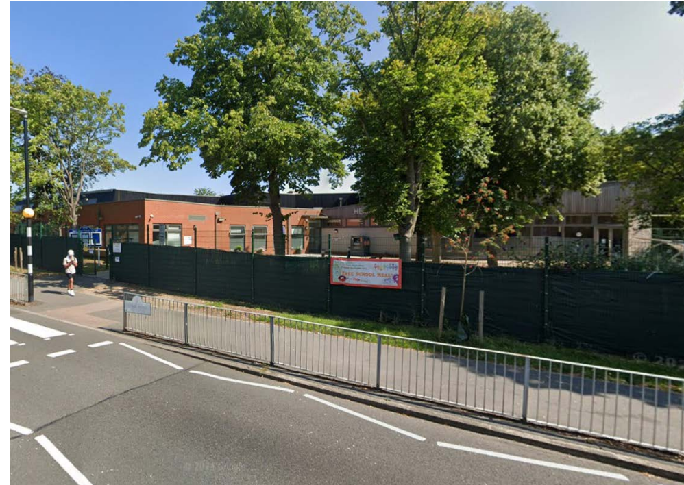
Figure 3.2 Hermitage Primary School, located on Belmont Road Source: Google Streetview July 2024
