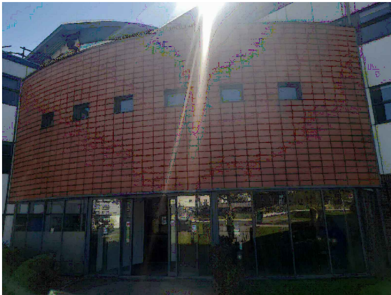
PHOTO A - EXISTING FRONT ENTRANCE
