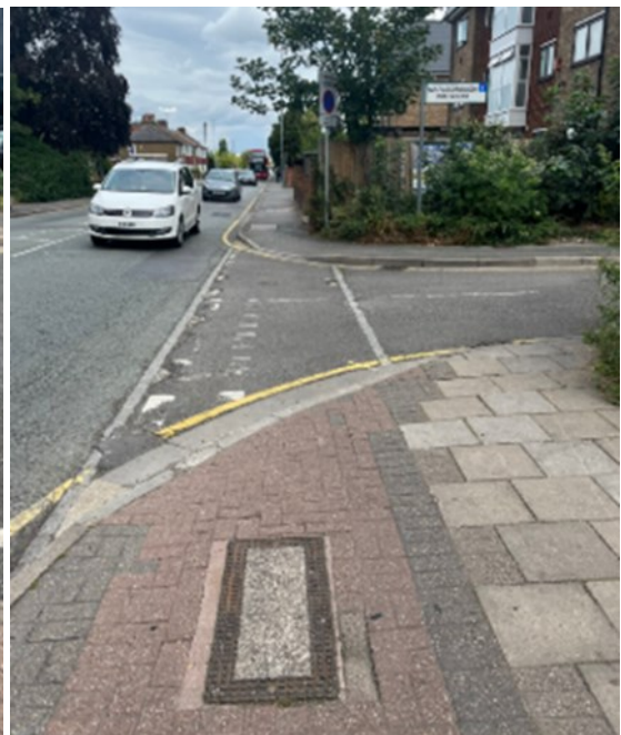
Photograph 3.7 (left): Dropped kerb pedestrian crossing across Nobel Drive looking west Photograph 3.8 (right): Dropped kerb pedestrian crossing across Marlborough Crescent looking north
