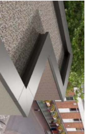
4. POWDER COATED (RAL 7016) ALUMINUM CAPPING TO PARAPETS
