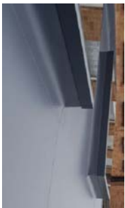
10. LIFT OVERRUN & SMOKE VENT (11.) Example of grey single ply roof upstands and details
