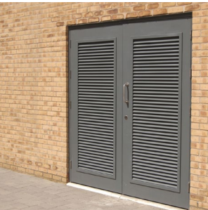
4. SERVICES DOORS: Dark grey - louvred for ventilation
