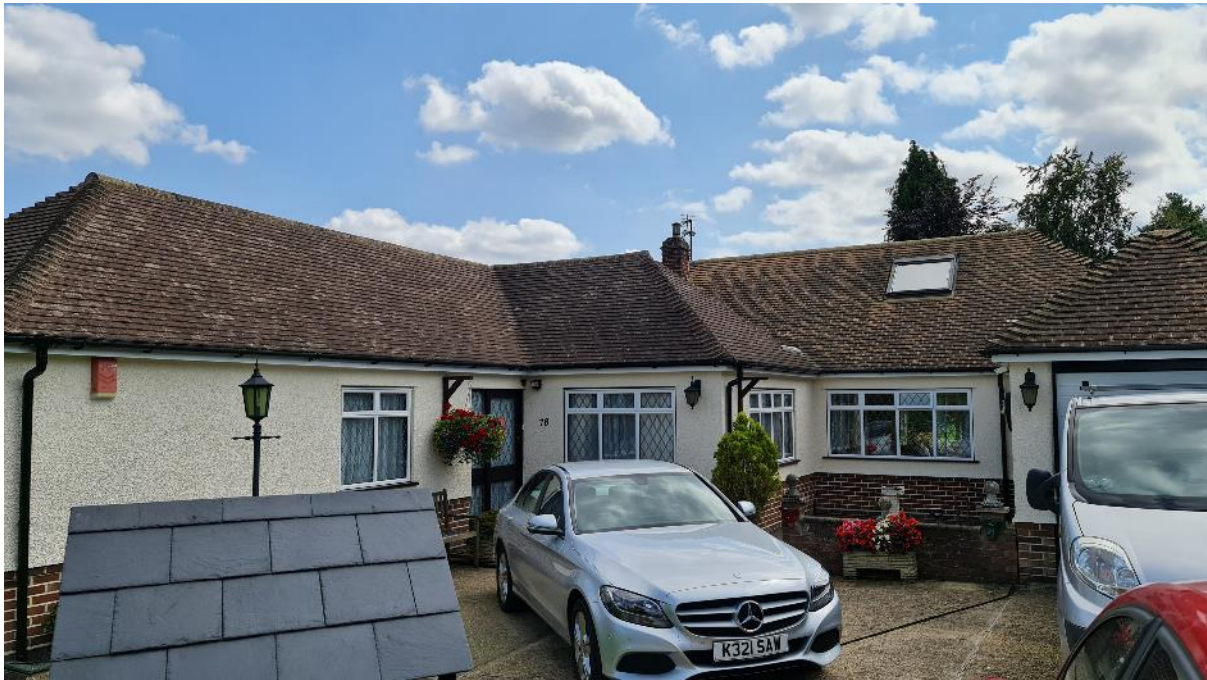
Figure 1: Northern elevation, facing south-east, with secure windows, doors and concrete tiled roof. Rendered brickwork appears in excellent condition.
