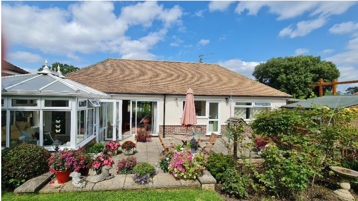
Figure 3: Southern elevation, with no damage to the rendering on the bricks, cracks or gaps. The soffits and fascia on the building are flush with no means of ingress and no evidence of bats. The roof tiles are in good condition, with no gaps, slipped or missing tiles. The conservatory is well-sealed too with no means of ingress.
