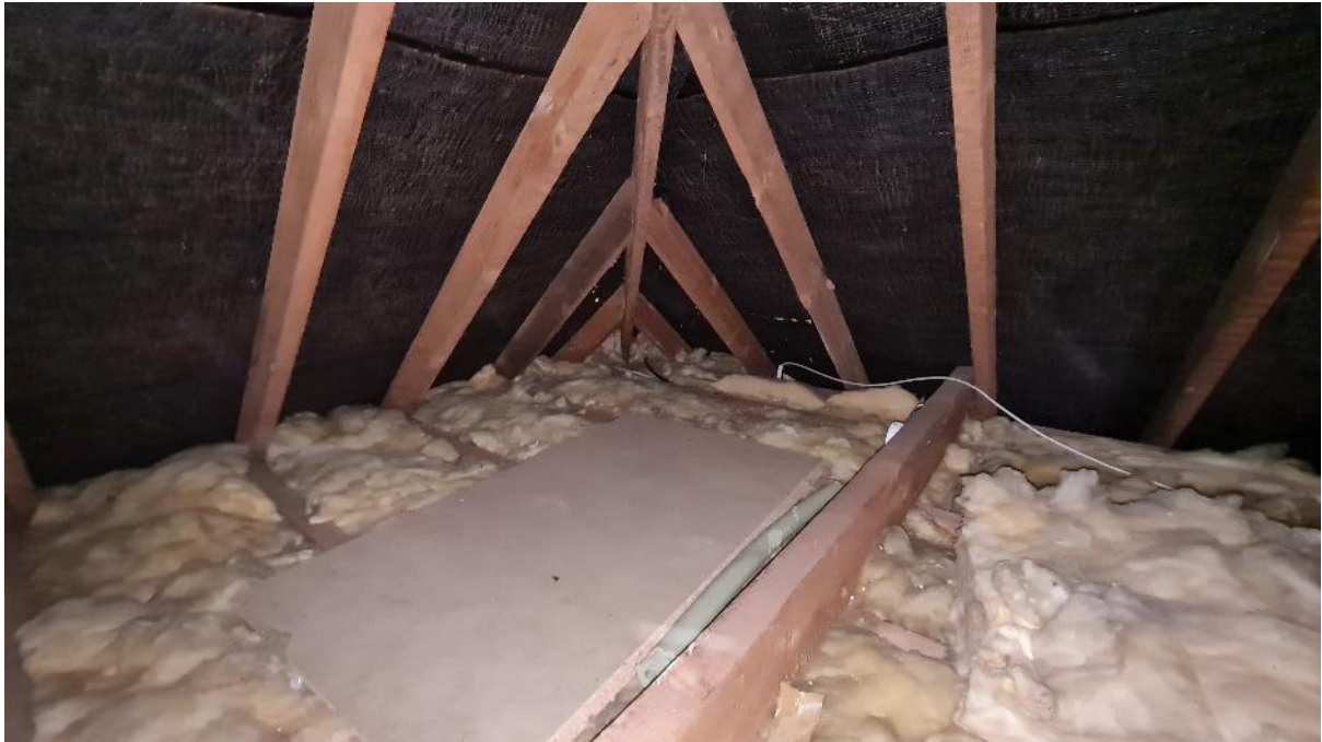
Figure 7: Loft space L1. Some boards for access and roll insulation across the loft space. Modern timbers present and black membrane lining the roof. There are cobwebs on the ridge of the loft space, no light entering from outside and no evidence of bats observed.
