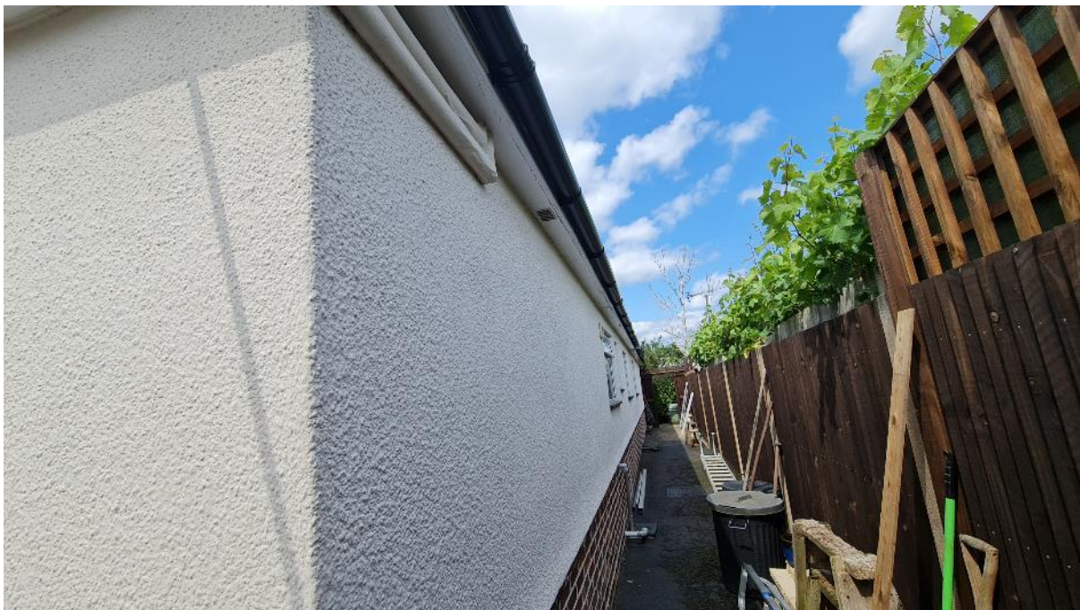
Figure 2: Eastern elevation with UPVC soffits and fascia in good condition, in addition to the rendered brickwork which appears to be in excellent condition with no gaps or cracks.
