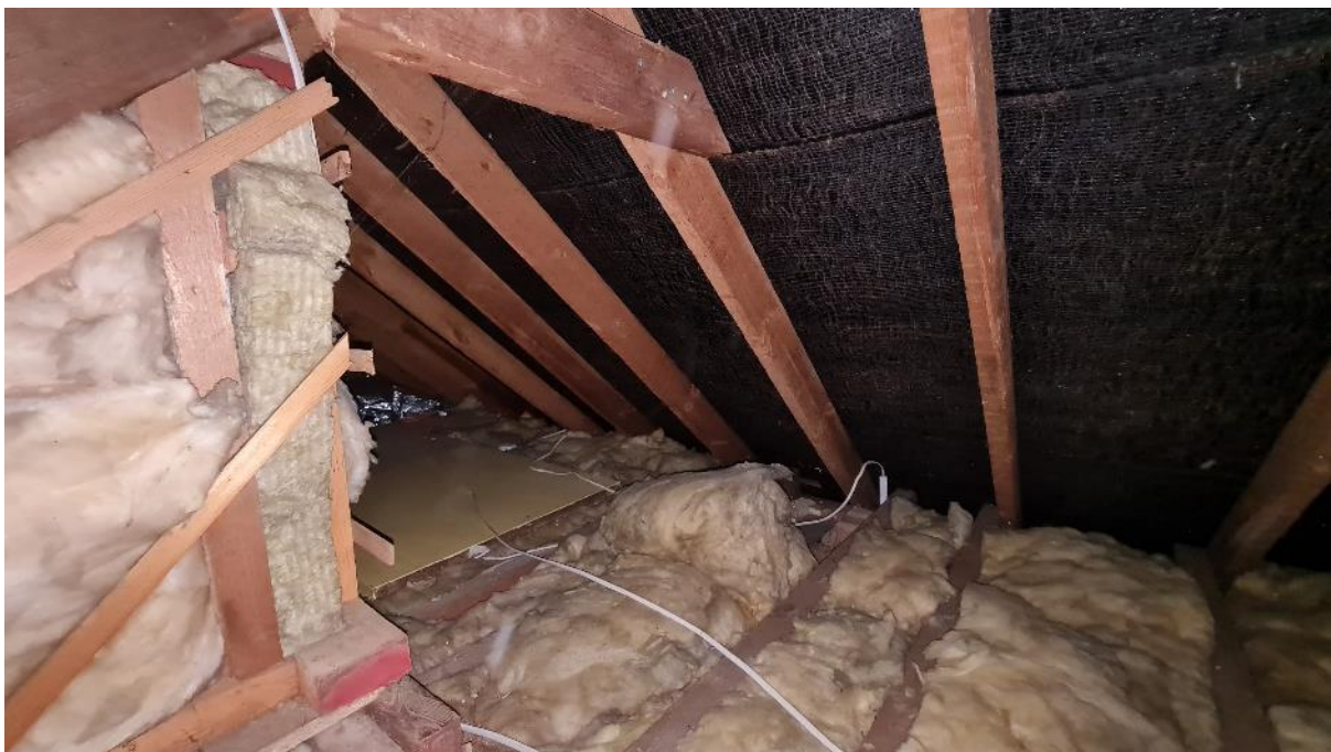
Figure 6: Loft space L1. Some boards for access and roll insulation across the loft space. Modern timbers present and black membrane lining the roof. There are cobwebs on the ridge of the loft space, no light entering from outside and no evidence of bats observed.
