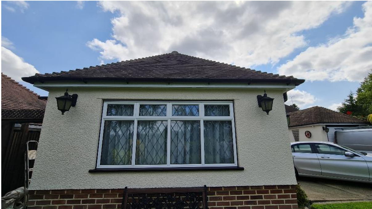
Figure 5: Northern elevation, with secure rendering on the brickwork, secure windows, and tiles all appear to be in good condition.
