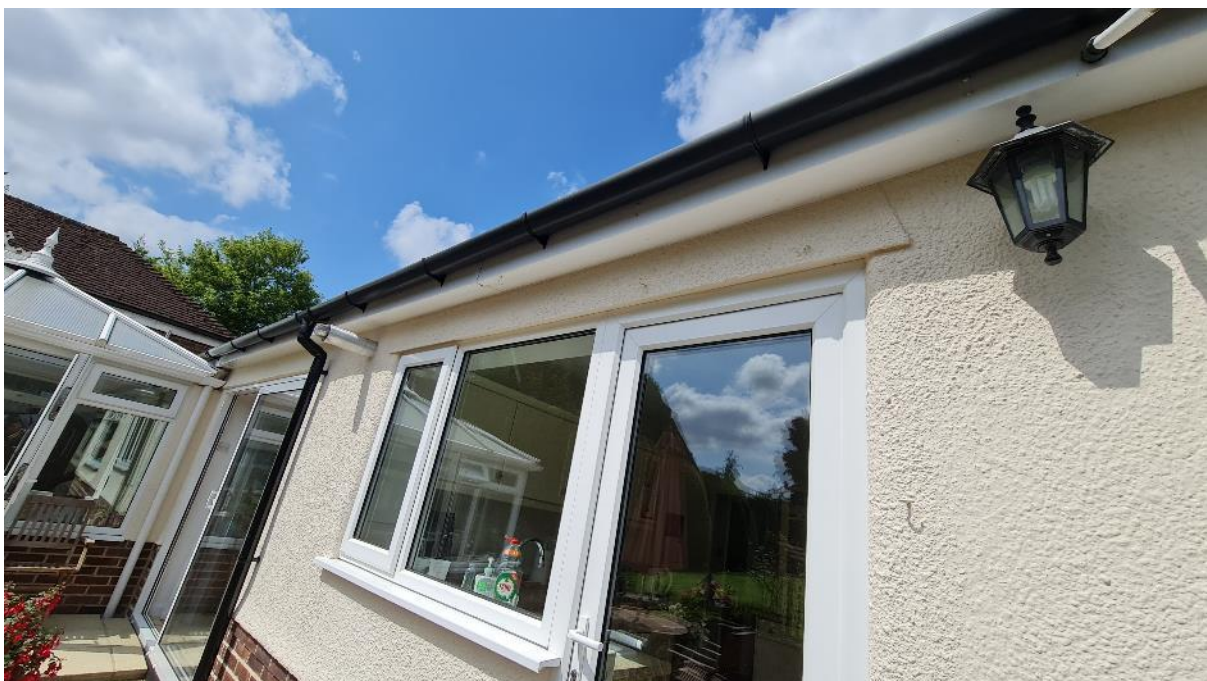
Figure 4: The UPVC windows, doors, soffits and fascia all appear to be in good condition with no gaps or means of ingress.
