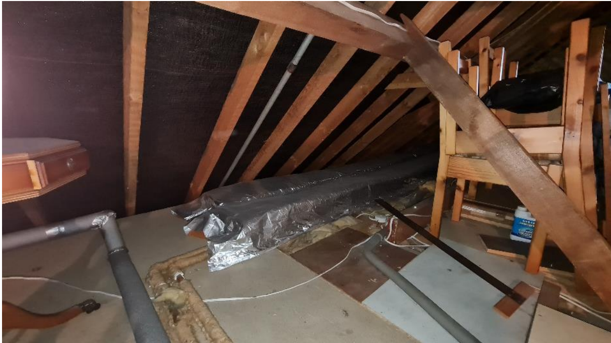
Figure 9: Loft space L2. Cobwebbing on the ridge beam and hanging from the modern timber beams. Black membrane lining the roof appeared to be in good condition with no gaps.
