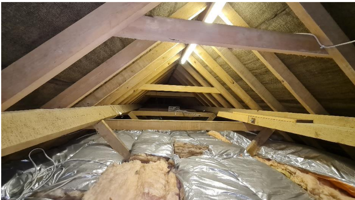
Figure 12: Loft space L2. This section of the loft (the most north-eastern section of the building) is the most modern with new timbers, unripped lining and new insulation present. There was no evidence of bats present within the loft.
