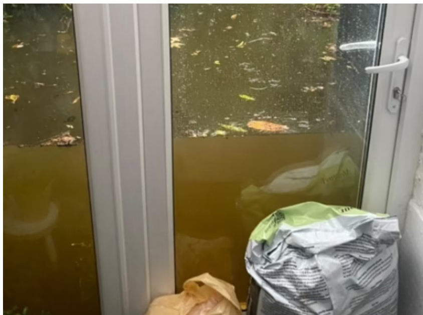
Figure 11: UPVC doors under flood conditions. These appear to offer reasonable flood resilience
