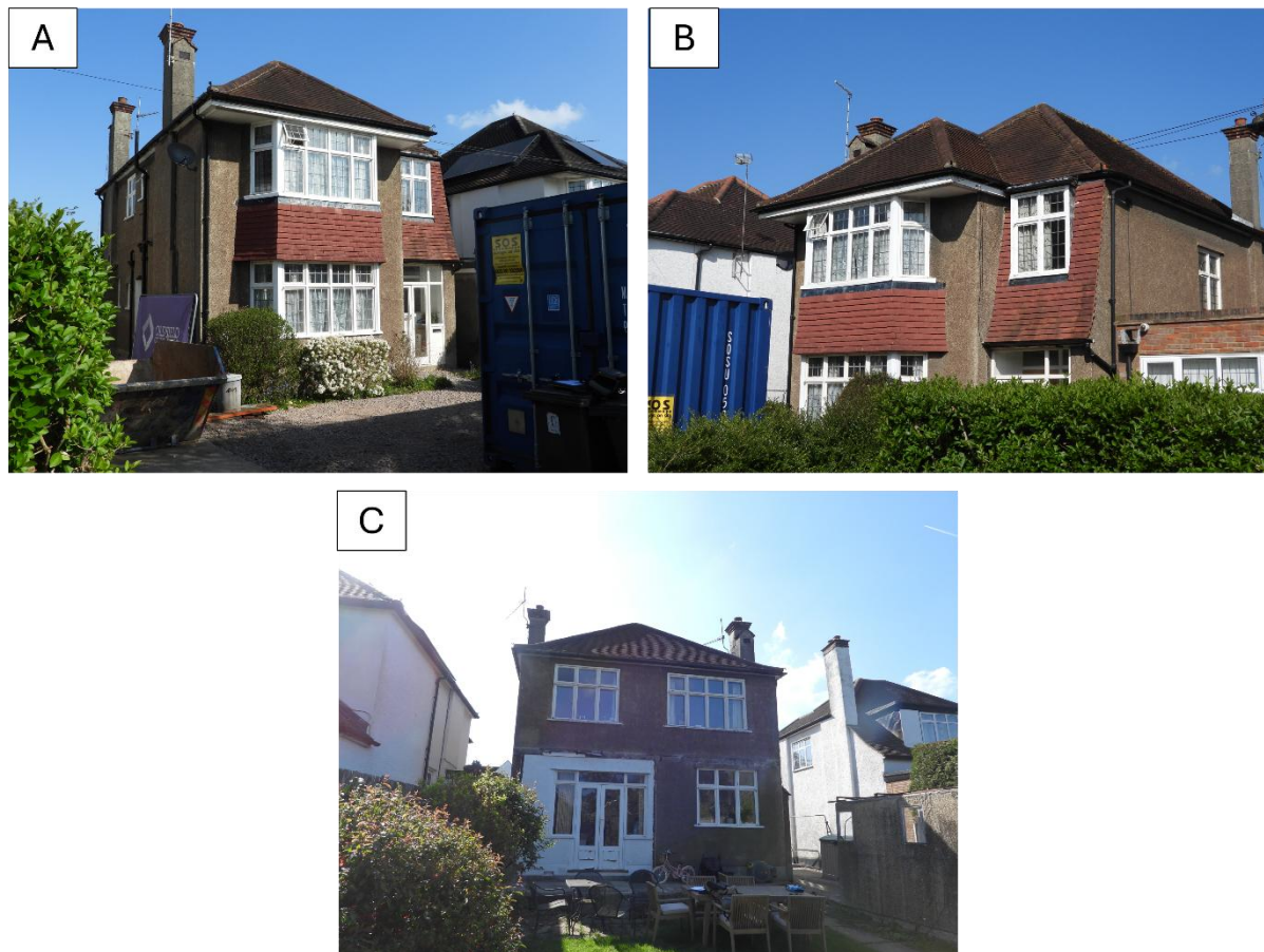
Figure 2: A) Southern western façade, B) South eastern façade, C) Northern façade
