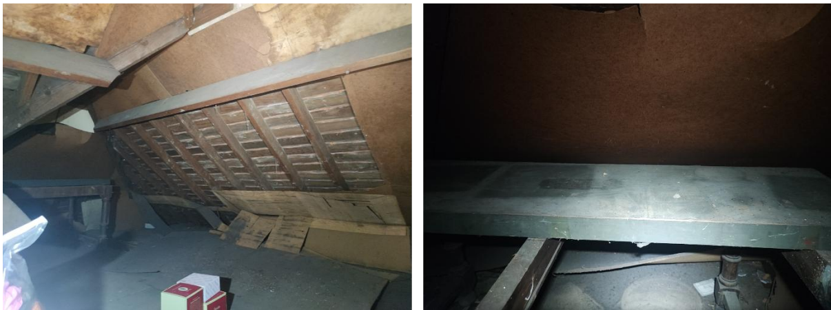
Figure 8: View of internal loft space at 98 Evelyn Ave Ruislip
