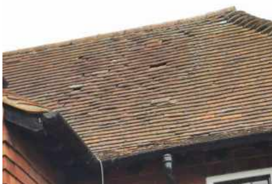
Photo 3. Suitable roosting features and access points for bats on Building 1.
