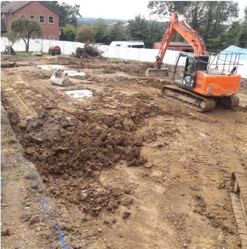
Photograph 1.1: Looking south west from south west corner of proposed building showing the strip and reduced level excavations carried out. With arisings removed from site.
