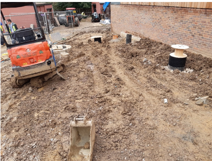
Photograph 1.3: Southern area of the site taken week commencing 12 th October 2020 showing the reinstatement of soils up to level in readiness for topsoil covering (100-150mm). Looking north west from the southern end of the site showing the south west corner of the new building (over the position of TP1).
