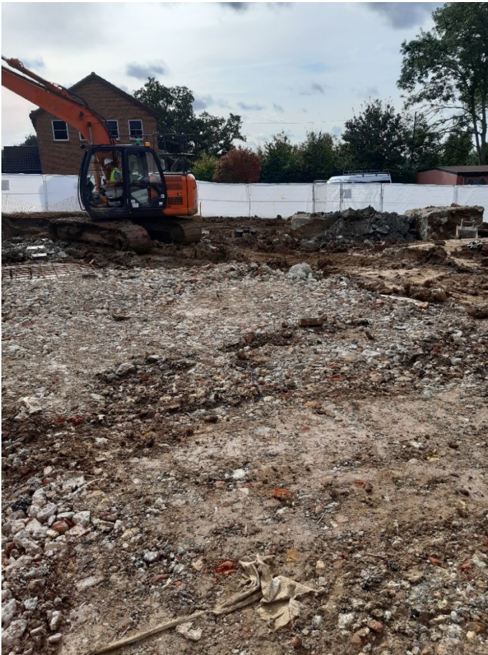
Photograph 1.2: Looking south west from south west corner of proposed building showing reduced level and imported working platform placed.
