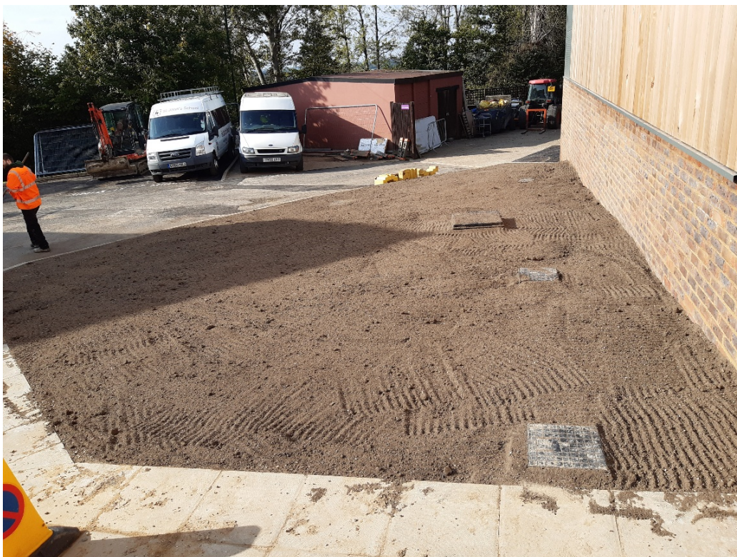
Photograph 1.4: Taken 19 th October 2020 showing placed imported topsoil in subject area
