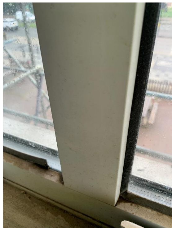
Image 3 Existing PVCu Windows
