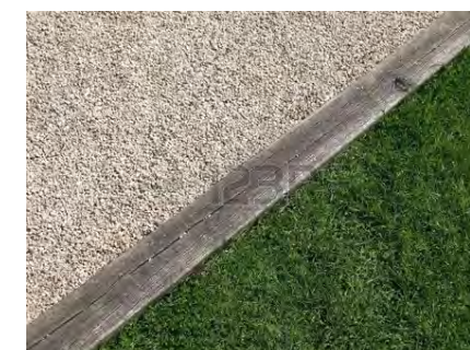
Figure 68 - timber edging to footpaths
