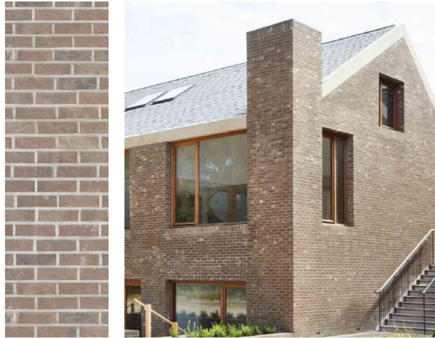
Light Brown Facing Brickwork
