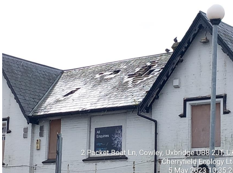
Figure 9: Holes shown in the exterior, with potential access to the space between the tiles and the lining
