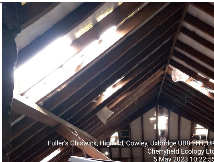
Figure 8: Further example of holes in roof
