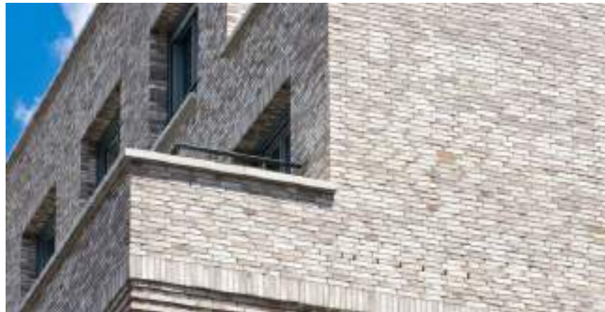
Flat parapets with set backs and soldier course banding.
