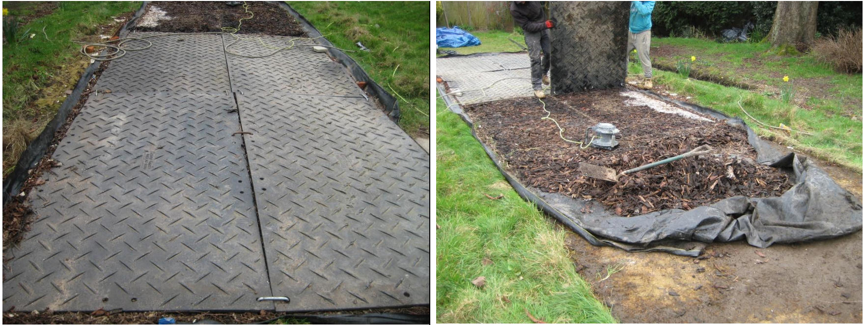
Fig 12 – Temporary ground protection is an effective way of allowing access through the RPA of retained trees. It must be installed prior to any on site activity and maintained for the duration of all works to be effective. Above left Tamla Trees project ground protection in place and above right being removed following the completion of site works. (Note: depending on the length of time it is in place it will adversely affect underlying grass ground cover which will need reseeded/ turfed accordingly)
