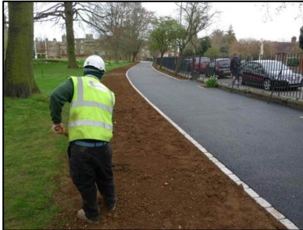
Fig 16 – All 'making good' topsoil will be BS3882 compliant and raked out by hand to no greater depth than 100mm.
