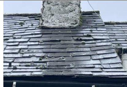
Figure 3: raised tiles on W. elevation
