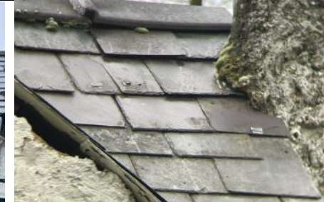
Figure 4: raised tiles on S. elevation
