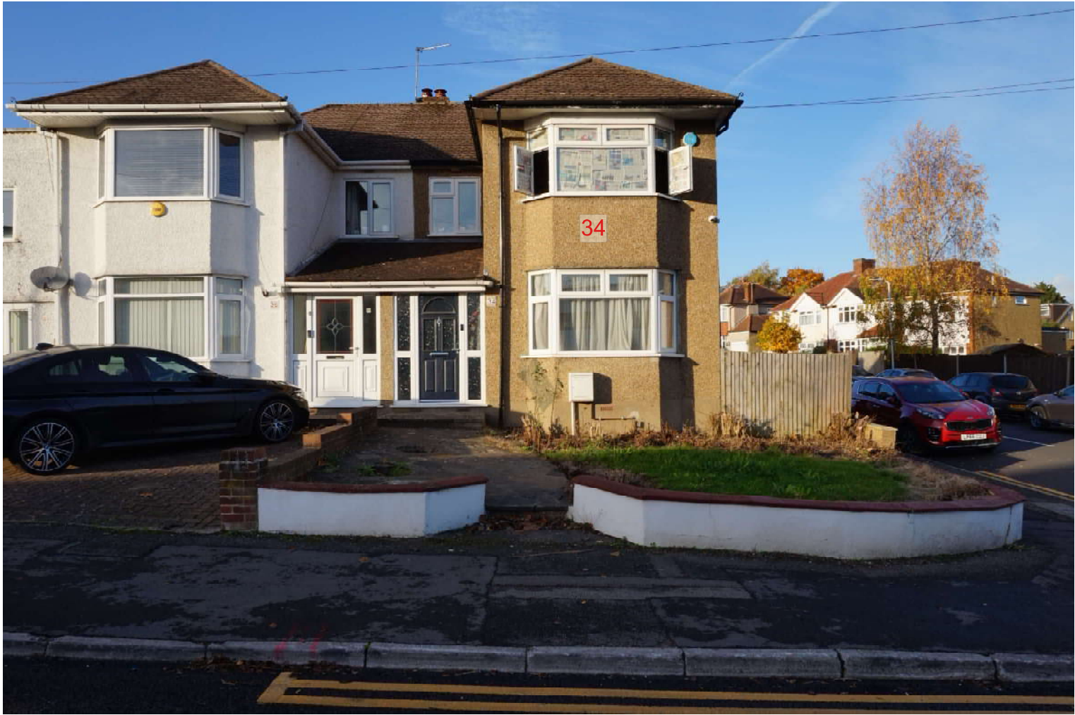
VIEW - FRONT (STREET)
